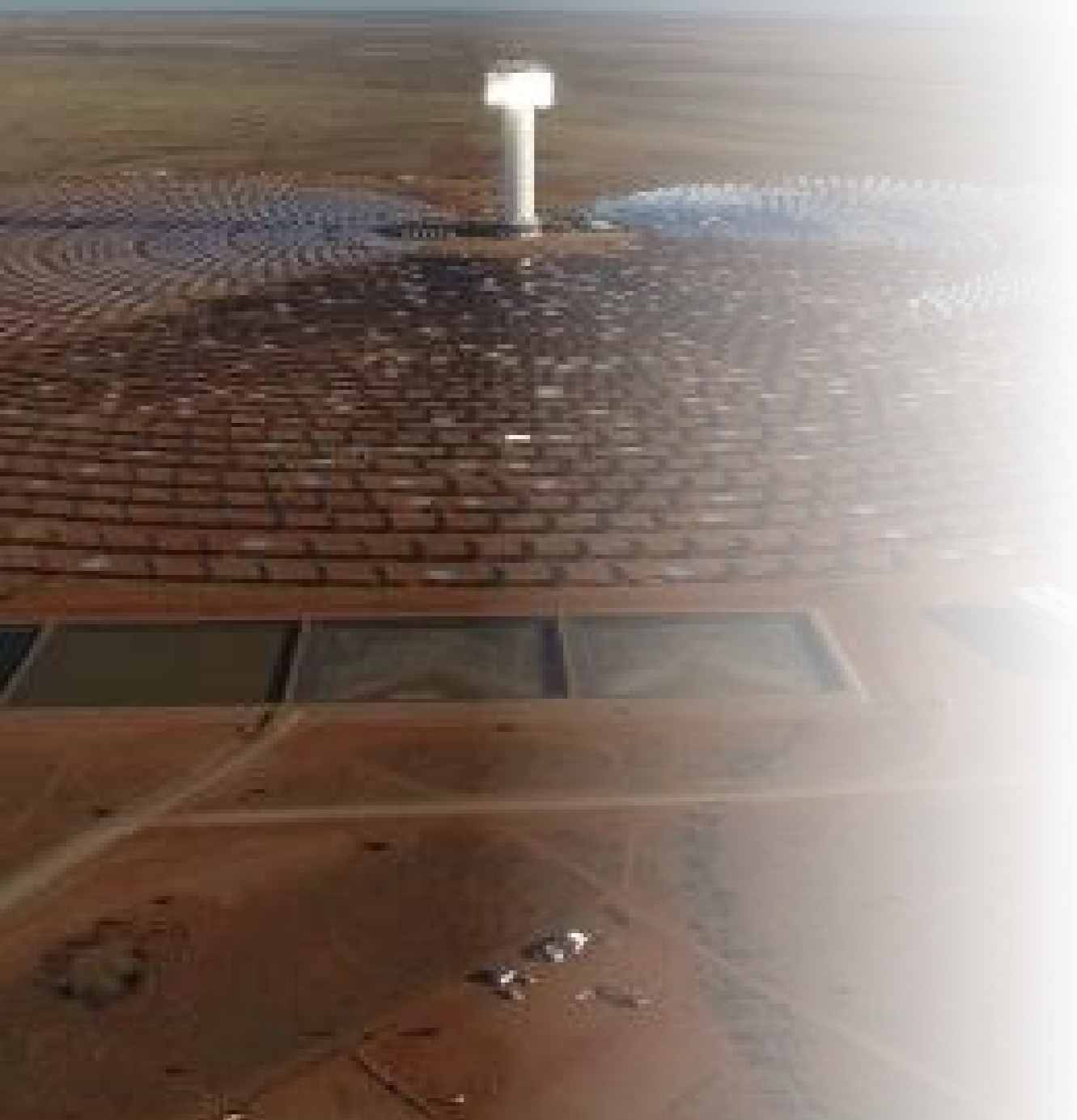
Khi Solar One solar thermal tower plant. 50 MW (South Africa)
