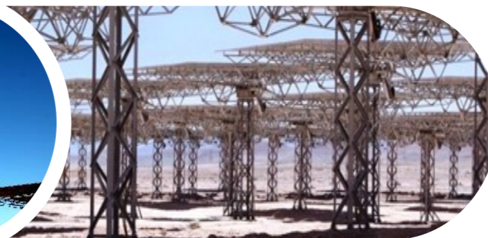
Cerro Dominador PV plant (Chile) – 10.600 uts
