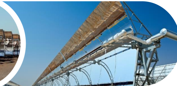
Shams Solar CCP (EAU) – 384 uts
