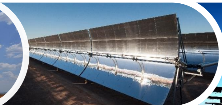
Ashalim Solar CCP (Israel) – 1344 uts
