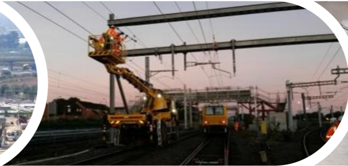
Electrificación Greater Western Region y Southern Region (UK)
