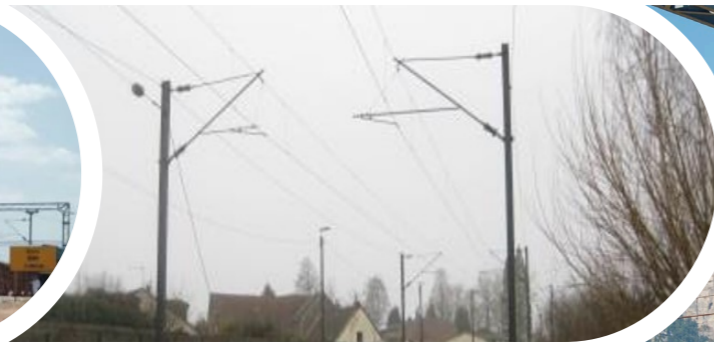
Renovation of catenary Landas-Valenciennes (France)
