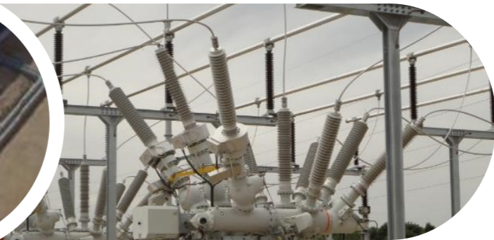
132kV Hybrid SS Pabellones (Spain)
