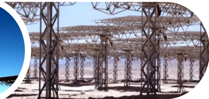
Cerro Dominador PV plant (Chile) – 10,600 uts
