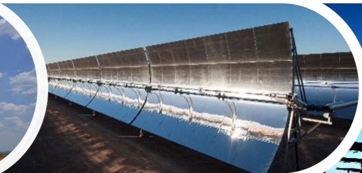
Ashalim Solar CCP (Israel) – 1344 uts
