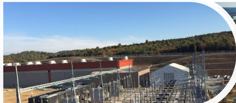
ITER (International Thermonuclear Experimental Reactor) (France)
