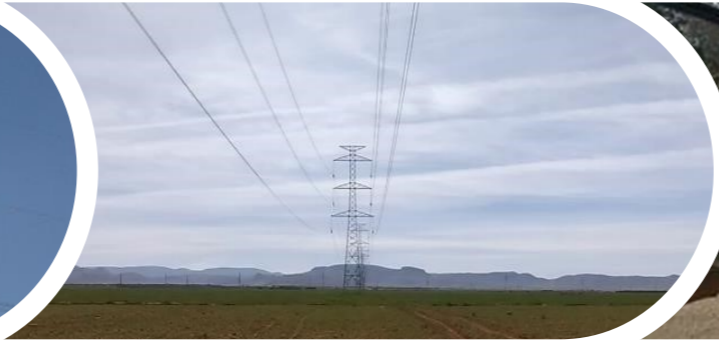
400kV TL Bourdim – Jerada (Morocco) – 12,000 Ton
