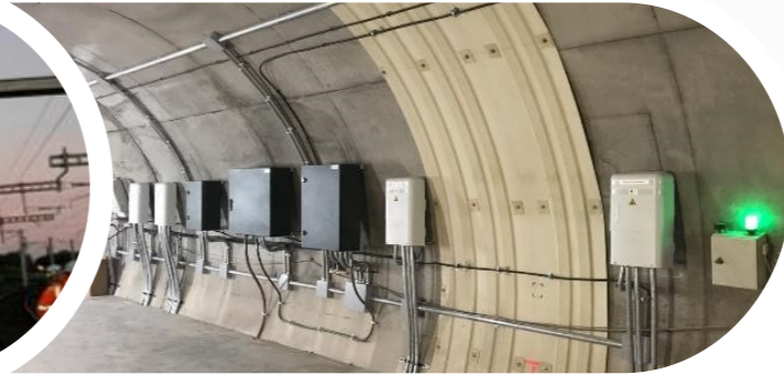
Communication and security systems HS La Robla-Pola de Lena (Spain)
