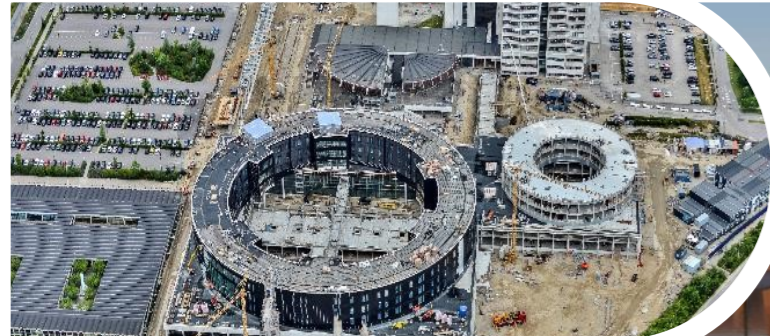
Herlev Hospital (Denmark)
