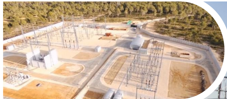
225/63 kV SS Castellet (France)
