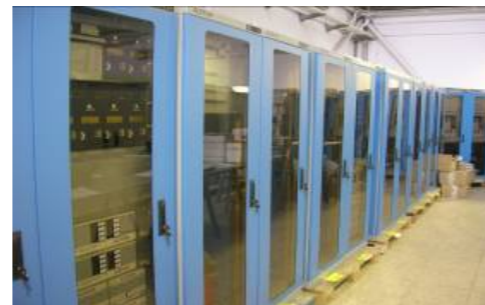
Control panels, Jerusalem tram for Alstom Transporte
