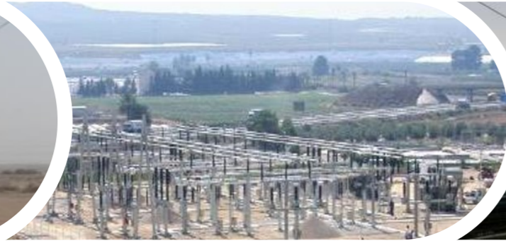
High speed lines - Catenaries & SS (Spain)
