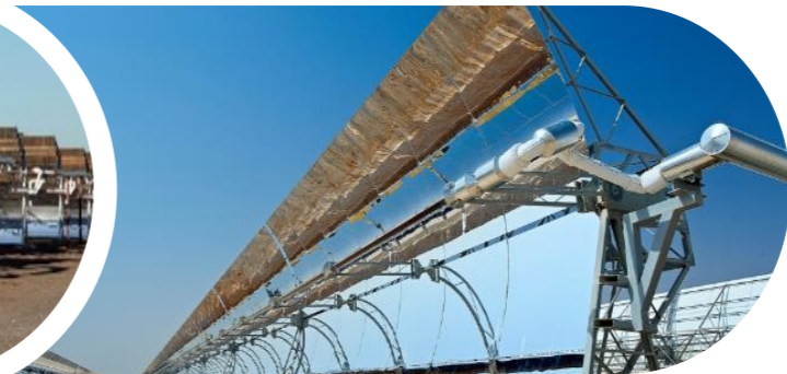
Shams Solar CCP (UAE) – 384 uts
