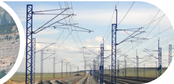
Maintenance HS Antequera-Granada (Spain)
