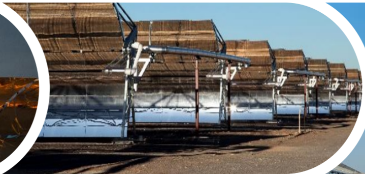
Kaxu Solar One CCP (South Africa) – 1,200 uts
