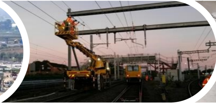
Greater Western Region y Southern Region Electrification (UK)
