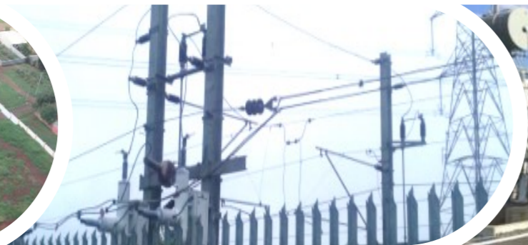
Beaulieu 400/55 kV Traction SS (UK)
