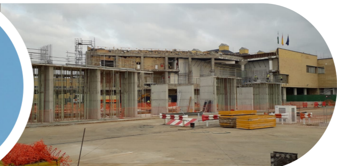
Remodeling of the passenger terminal at Seville Airport (Spain)
