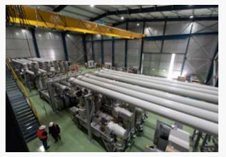
The 345 kV Altiplano switching station, with AIS and GIS technology and specific designs due to its location at 4,000 meters above sea level, became operational in 2020.
