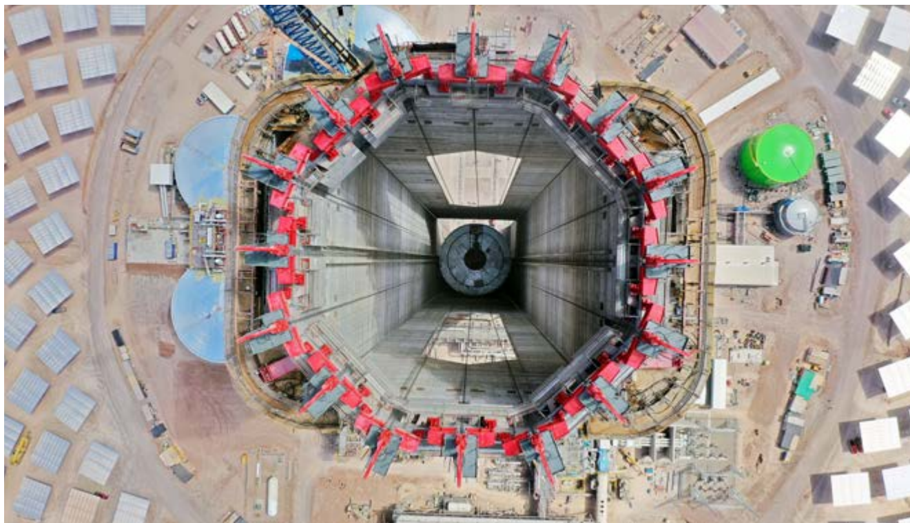
► Hoisting the receiver of the Cerro Dominador solar thermal plant.
