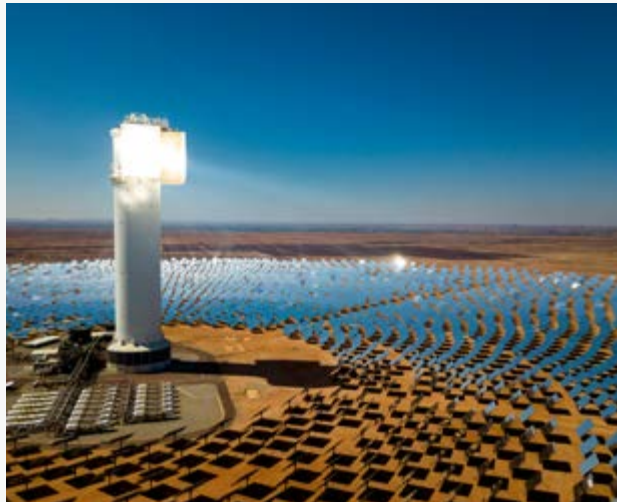
► The KHI Solar One solar thermal plant, built by Abengoa, is fully operational.
