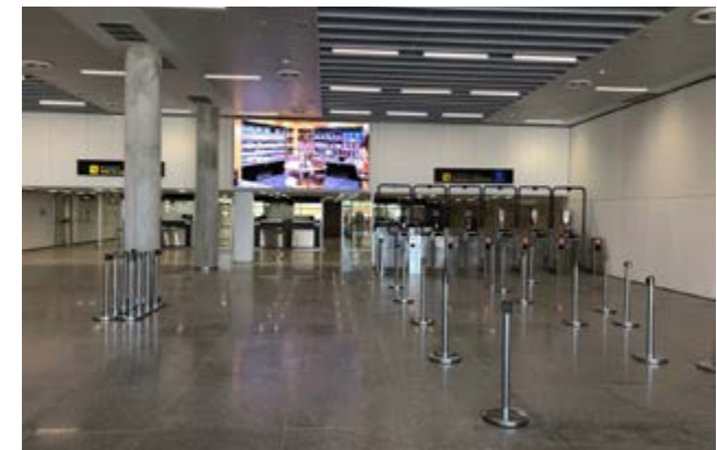
► Abengoa continues with the refurbishment and extension of the San Pablo Airport Terminal building in Seville (Spain).
