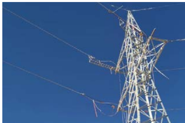
► Work on the evacuation line of a wind farm in Chile.
