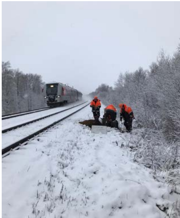
► Engineering works for the Vilnius-Klaipeda railway electrification project in Lithuania.
