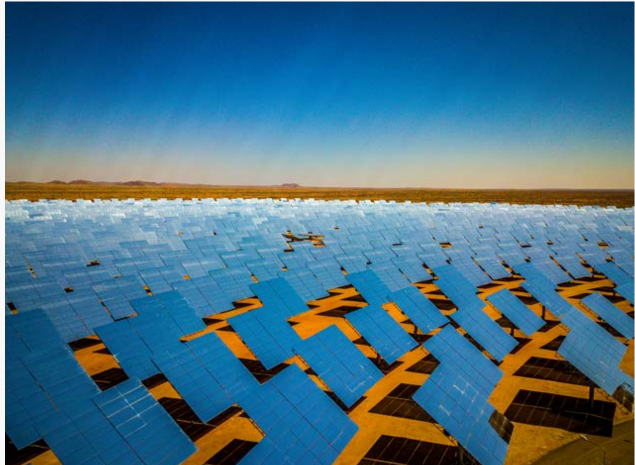
► View of the solar field from the Khi Solar One tower plant.
