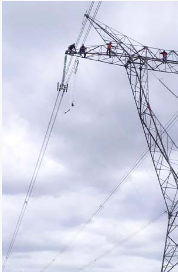
► Maintenance work on an existing 550 kV line.
