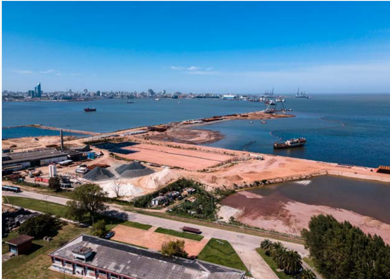
► Abengoa works at Puerto Capurro Fishing Terminal.
