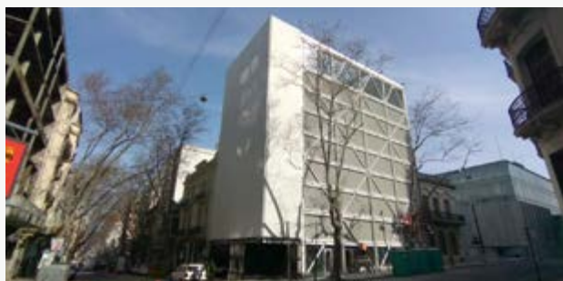
► In 2020, Abengoa completed the construction of a large parking lot in downtown Montevideo.
