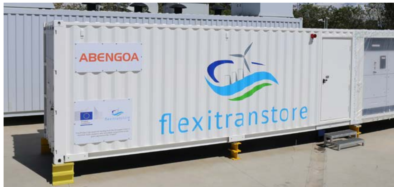
▶ The Flexitranstore project is designed to bring stability to the power supply using lithium ion batteries.
