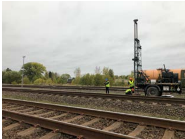
► Abengoa is an international leader in catenary, substation, communications and auxiliary installation activities.
