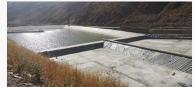
► 30,000 m 3 capacity retention dam reservoir built by Abengoa for the Cuajone mine.
