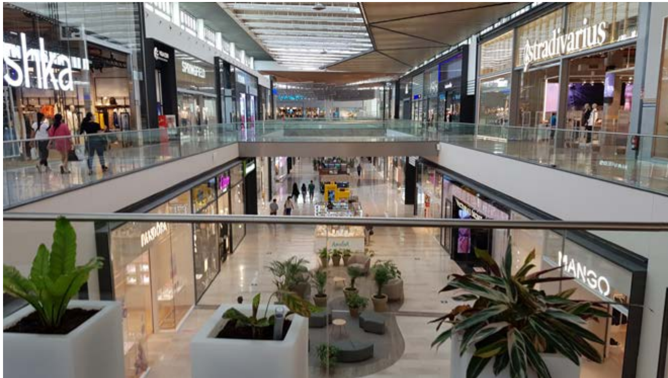
► Abengoa is responsible for the integral maintenance of the electromechanical installations of the Lagoh shopping and family leisure centre (Seville).
