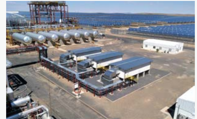
► Containers for the new Kaxu Solar One variable frequency drives.
