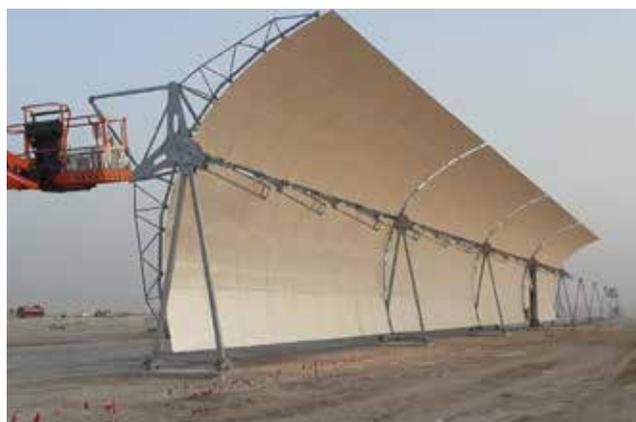
► One of the cylindrical-parabolic collectors of the solar field of stage IV of Al Maktoum Solar Park.
