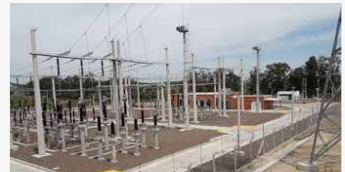
► Tacuarembó B power station with a capacity of 150 kV.
