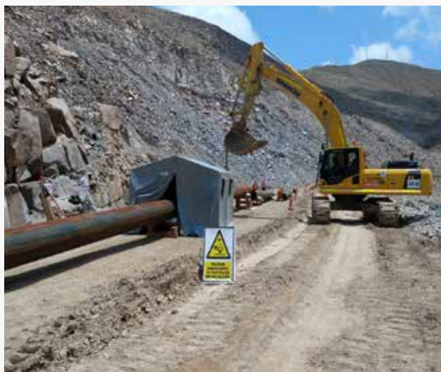
► Abengoa's works on the Incapuquio project in Toquepala.
