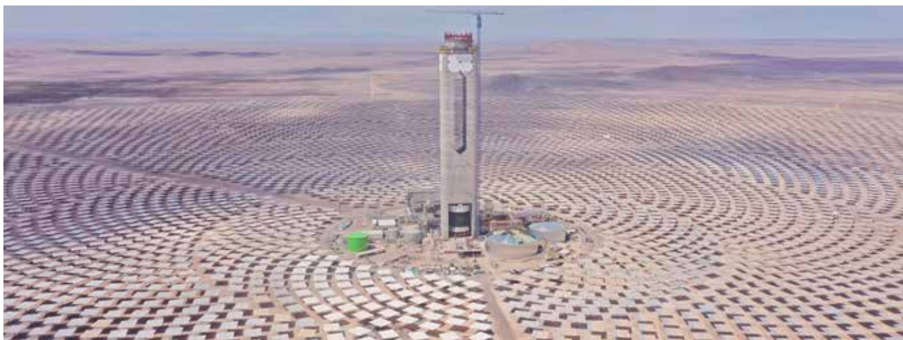
► Abengoa’s experience in renewable and conventional plants both in the construction and installation stages accumulates more than 12.8 GW.
