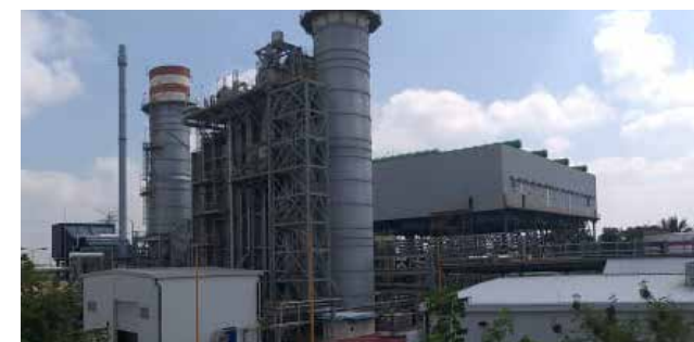
► A3T efficient cogeneration plant, in Mexico.
