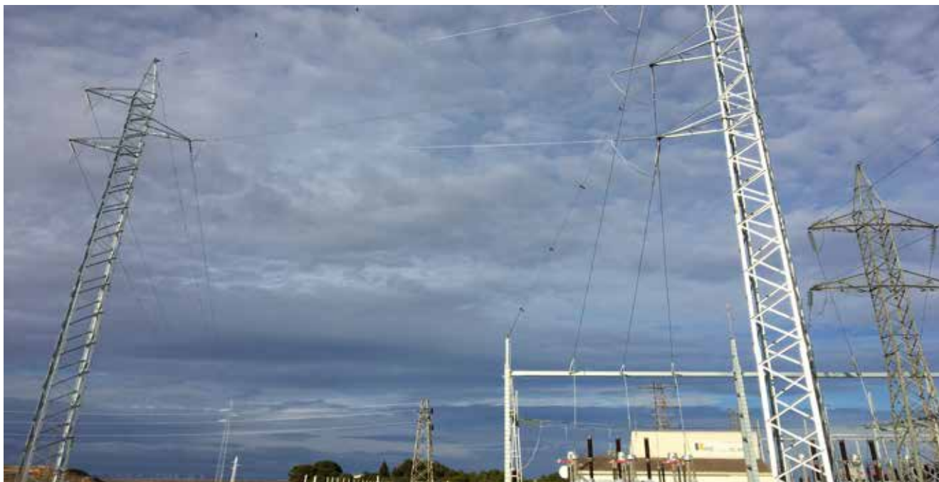
► A tower of our own design for the 132 kV San Agustín (Zaragoza) line manufactured by Eucomsa.
