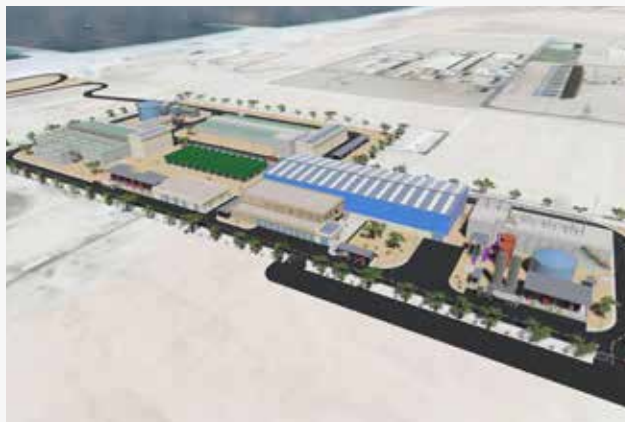
► Desalination plant in Salalah, Oman, which will operate with reverse osmosis technology and will have a capacity of 114,000 m 3 /day.
