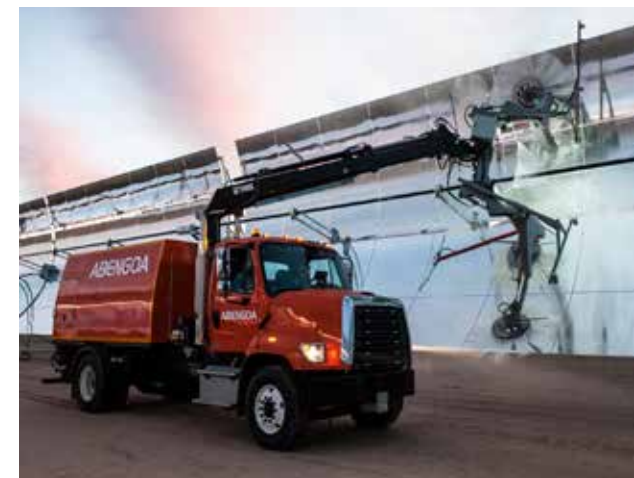
► Operation and maintenance work on a solar plant.
