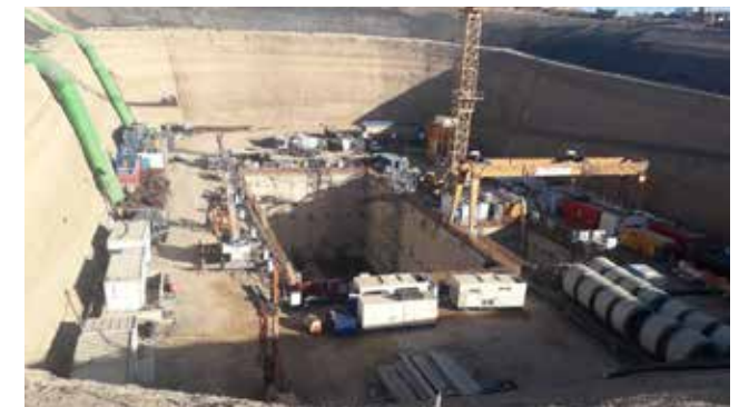
► Abengoa is constructing in Agadir (Morocco) a desalination plant with a capacity of 275,000 m 3 /day.
