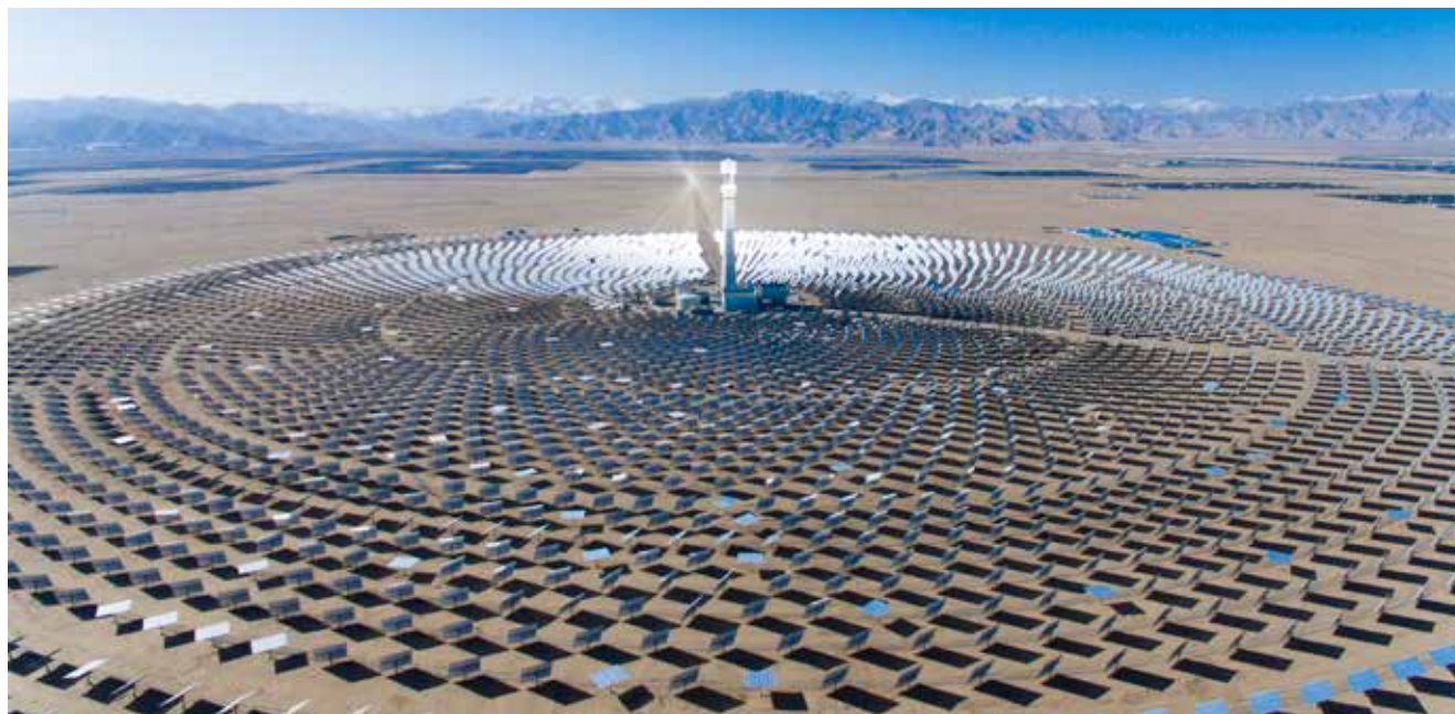
► Solar thermal tower plant of Luneng Haixi.
