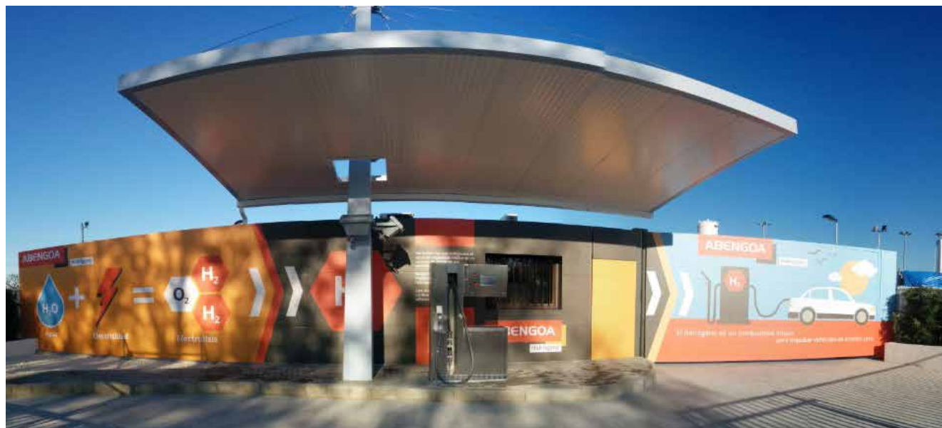
► Hydrogen service station.
