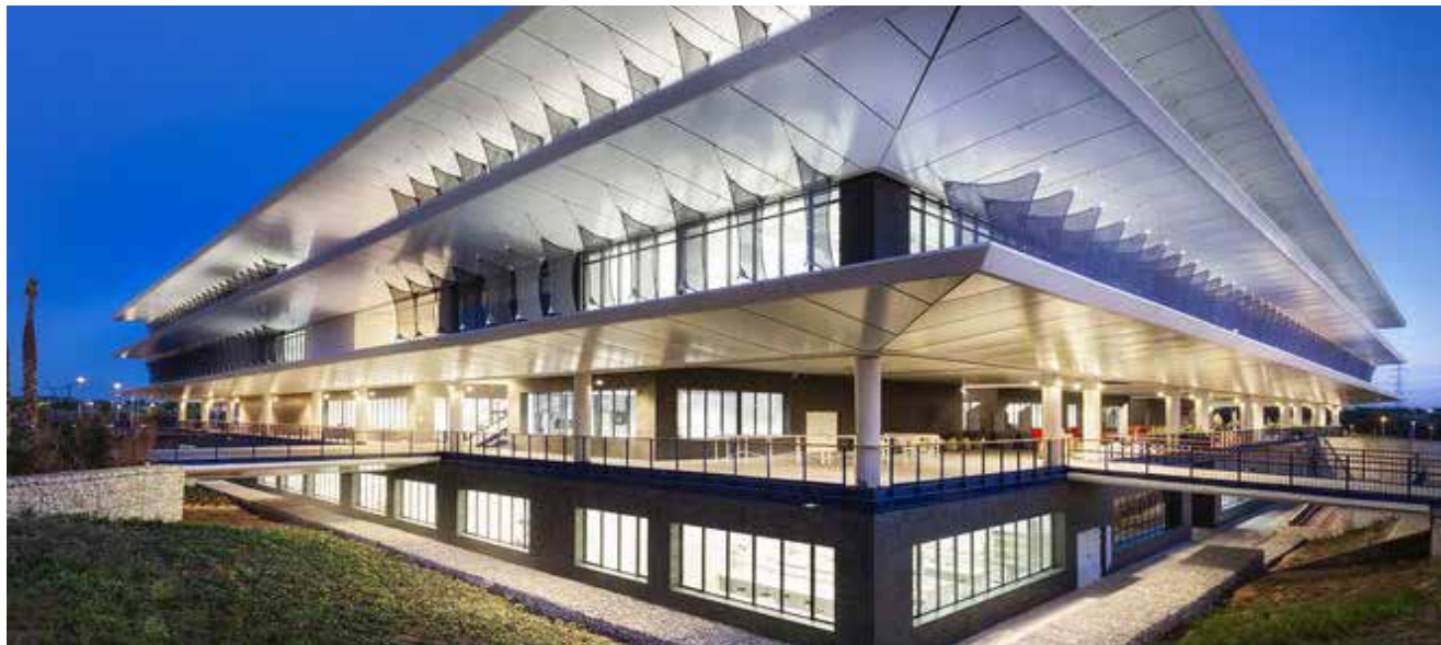
► In Spain, Abengoa has taken part in important infrastructure project all around the peninsula. In the image, the new headquarters of Universidad de Loyola in Dos Hermanas (Seville).
