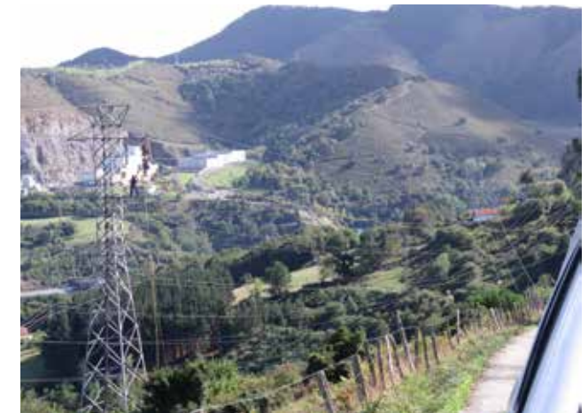
► Transmission line connecting Alonsotegi with Ortuela, in Biscay.
