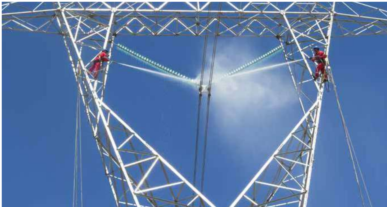
► Labour work and maintenance work on a transmission line.
