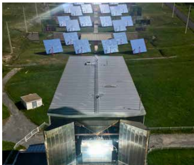
► Pilot plant of the Solpart project.
