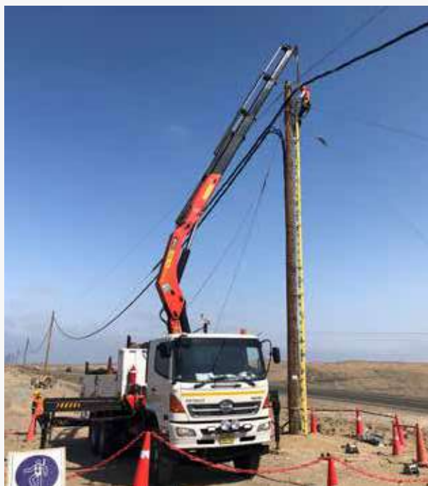
► Transmission line project from the port of Marcobre to the Mina Justa substation for Techint.
