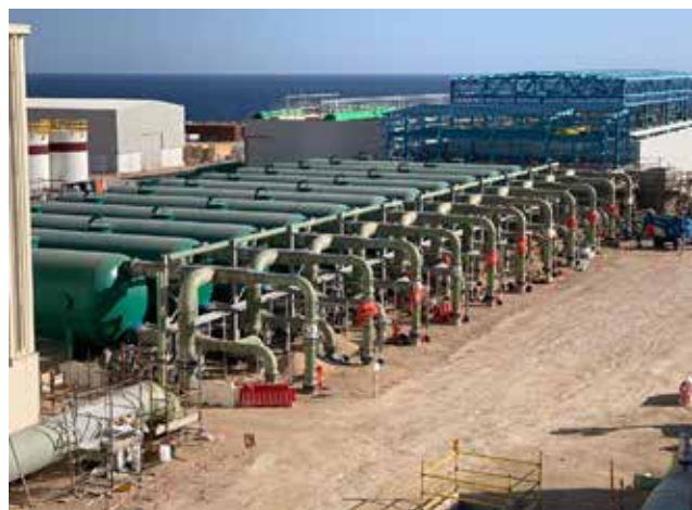
► Abengoa's desalination under construction in Salalah, Oman, will work with reverse osmosis technology.
