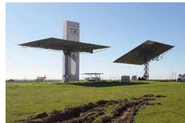
► Detail of heliostats in Pontones.
