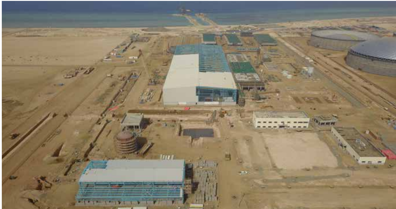
► Abengoa is leader in the water industry thanks to its large water desalination, purification and infrastructure. In the image, the works in the desalination plant of Rabigh (Saudi Arabia).
