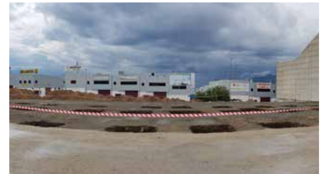
► Commencement of the works (cementation) of Mutua Universal in Málaga.
