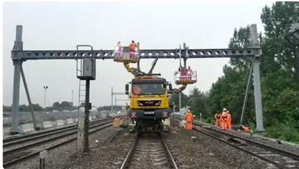
Overhead contact line work in the United Kingdom.
