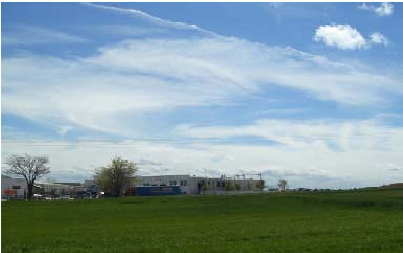
Industrial waste management center, Ajalvir, Spain
