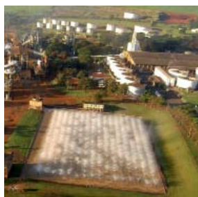
Bioethanol plant in Pirassununga, São Paulo, Brazil
