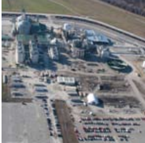
Bioethanol plant in Madison, Illinois
