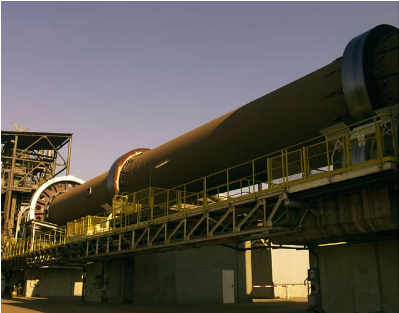
Waelz furnace in Erandio (Spain)
