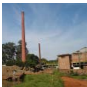
Sugar production plant in Santo Antônio de Posse, São Paulo, Brazil
