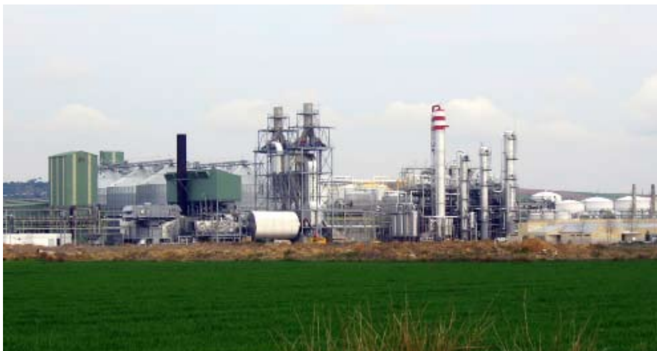
Bioethanol plant in Babilafuente, Salamanca
