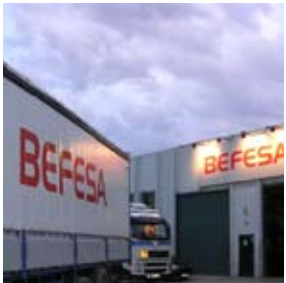
Waste management facilities in Ajalvir, Spain
