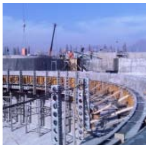
Construction of a liquid industrial waste treatment facility at the Quilicura plant in Chile
