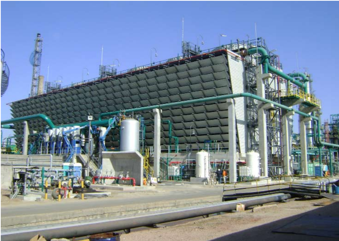
Desulfurization plant at La Teja Refinery
