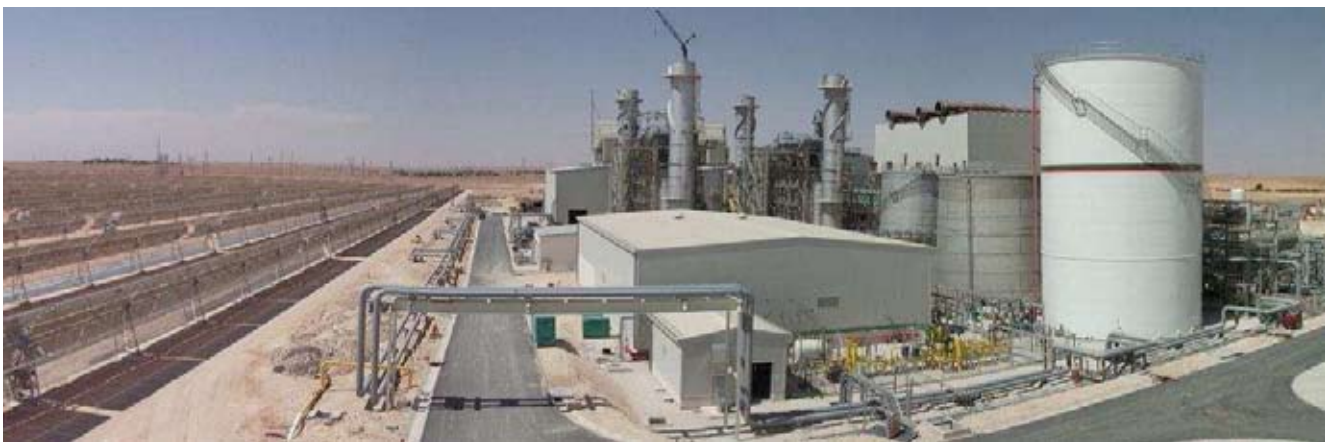
Hassi R'Mel ISCC plant in Algeria
