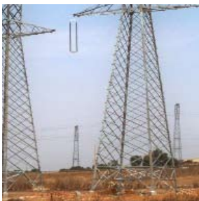
HV lines for the Moroccan motorway administrator
