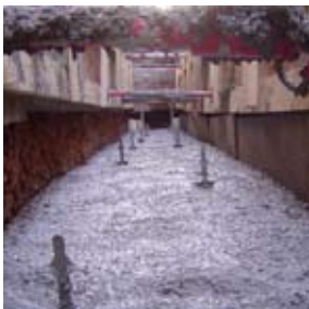
Ducting of high-voltage cables in Puigreig street, Barcelona
