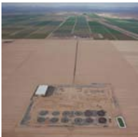
Overhead shot of ongoing construction work on the Solana plant
