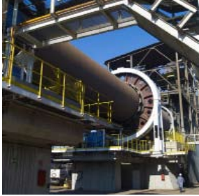
Waelz furnace in Erandio (Spain)
