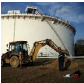
Abengoa employees performing soil decontamination work
