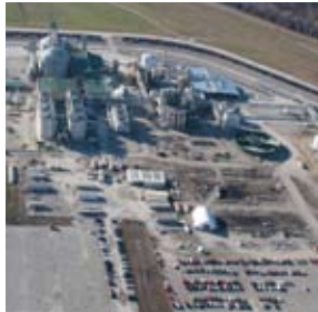
Bioethanol plant in Madison, Illinois
