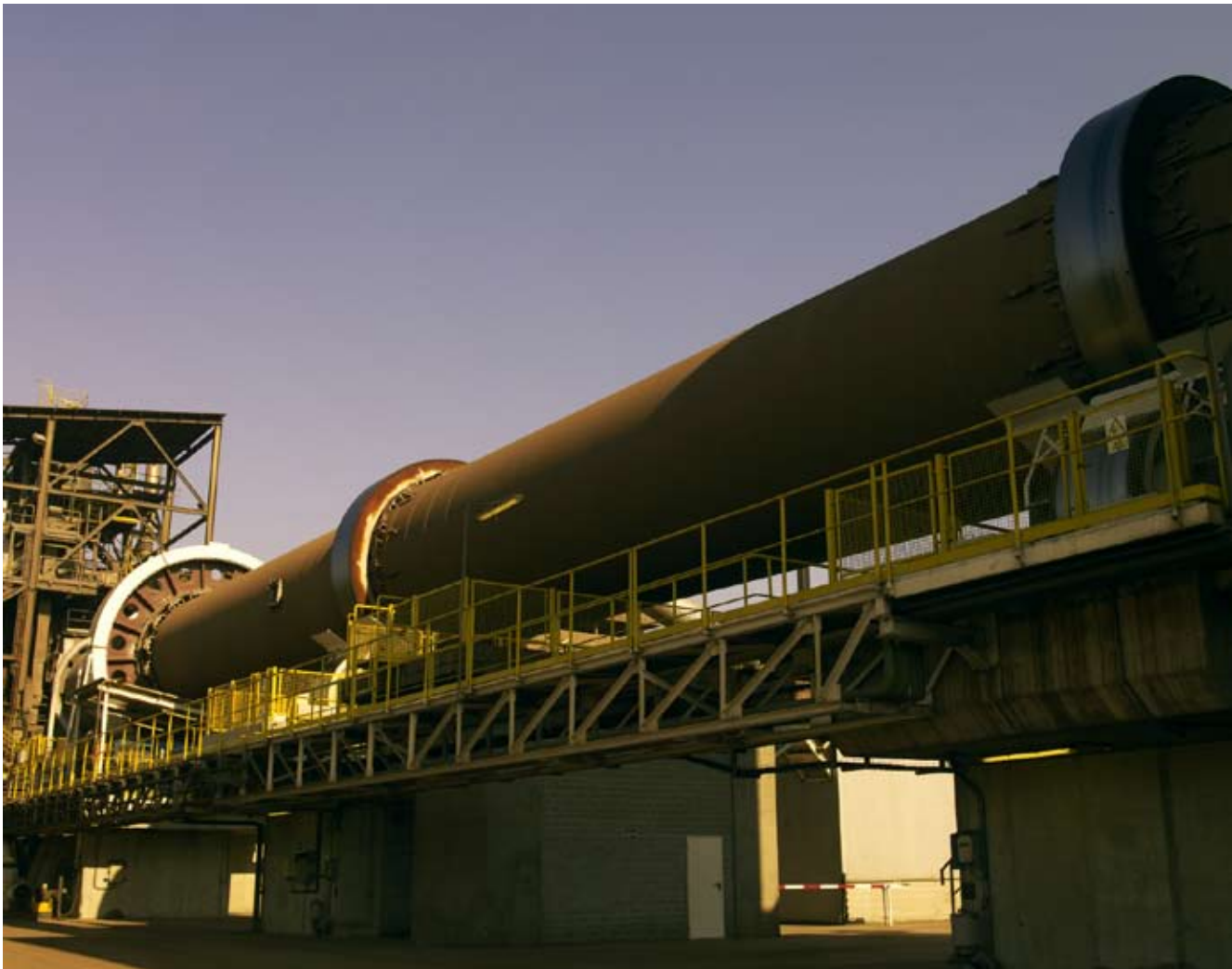
Waelz furnace in Erandio (Spain)
