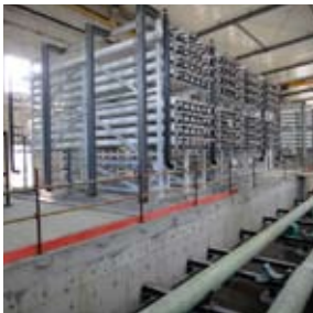
Osmosis racks at the Qingdao desalination plant in China
