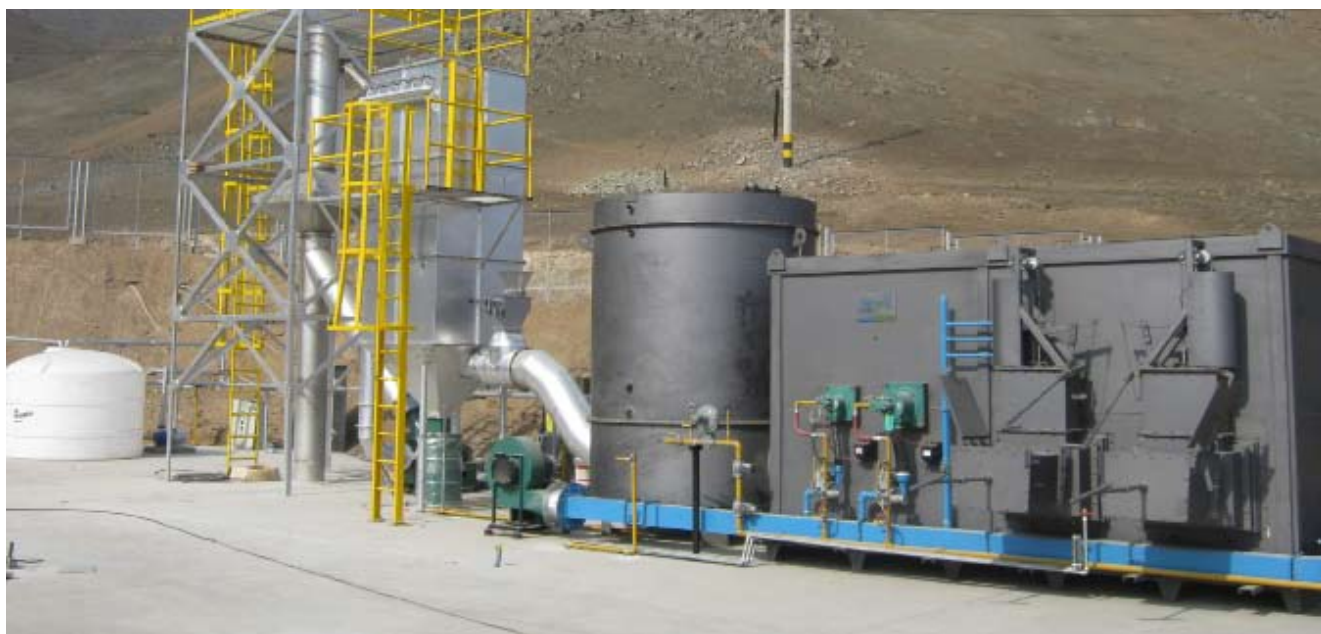
Peru's incinerator, the country's first facility of its kind
