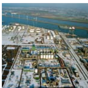
Bioethanol plant at the Europoort, Rotterdam, Holland
