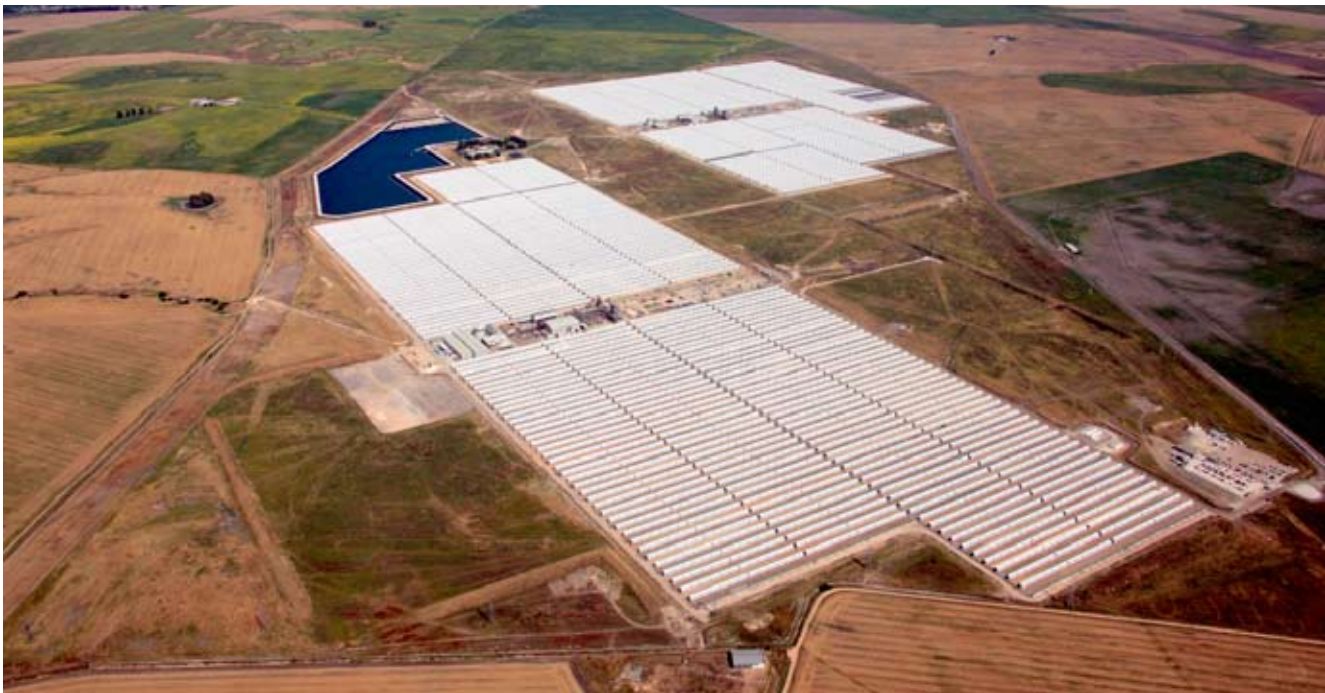
Helioenergy 1 and 2 in Ecija (Seville, Spain)
