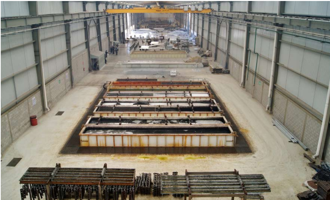
Workshop for galvanized structures
