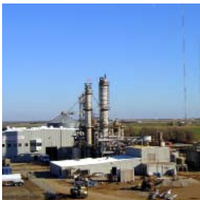
Bioethanol plant in Colwich, Kansas
