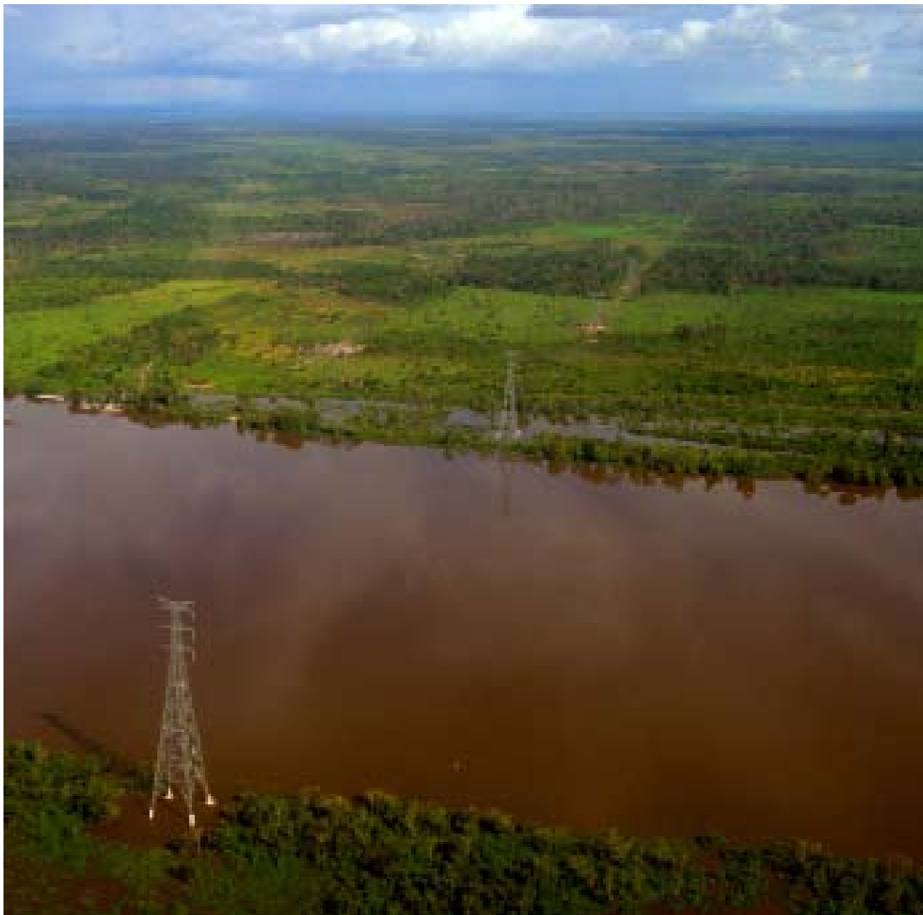
ATE III 230 kV transmission line crossing the river Araguaia (Brazil)
