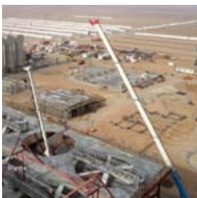
100 MW CSP plant in Abu Dhabi.
