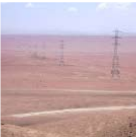
220 kV transmission line between Montalvo and Tía María, Peru
