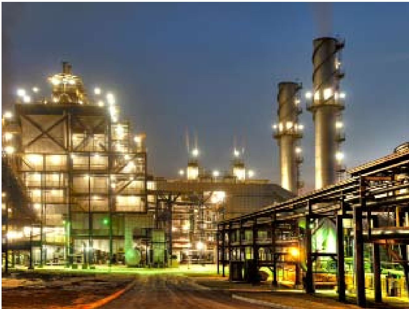
Cogeneration at the plant located in São Luiz, Pirassununga, Brazil
