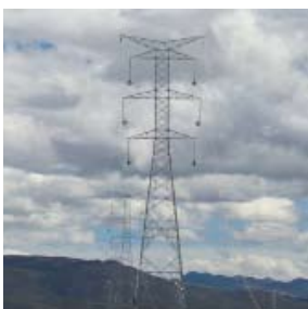
220 kV Carhumayo-Cajamarca transmission line
