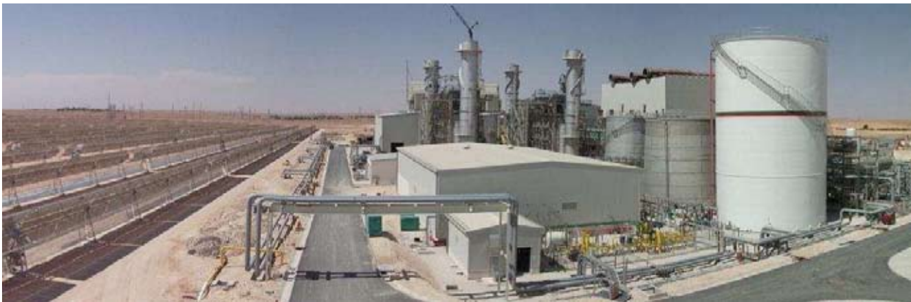
Hassi R'Mel ISCC plant in Algeria
