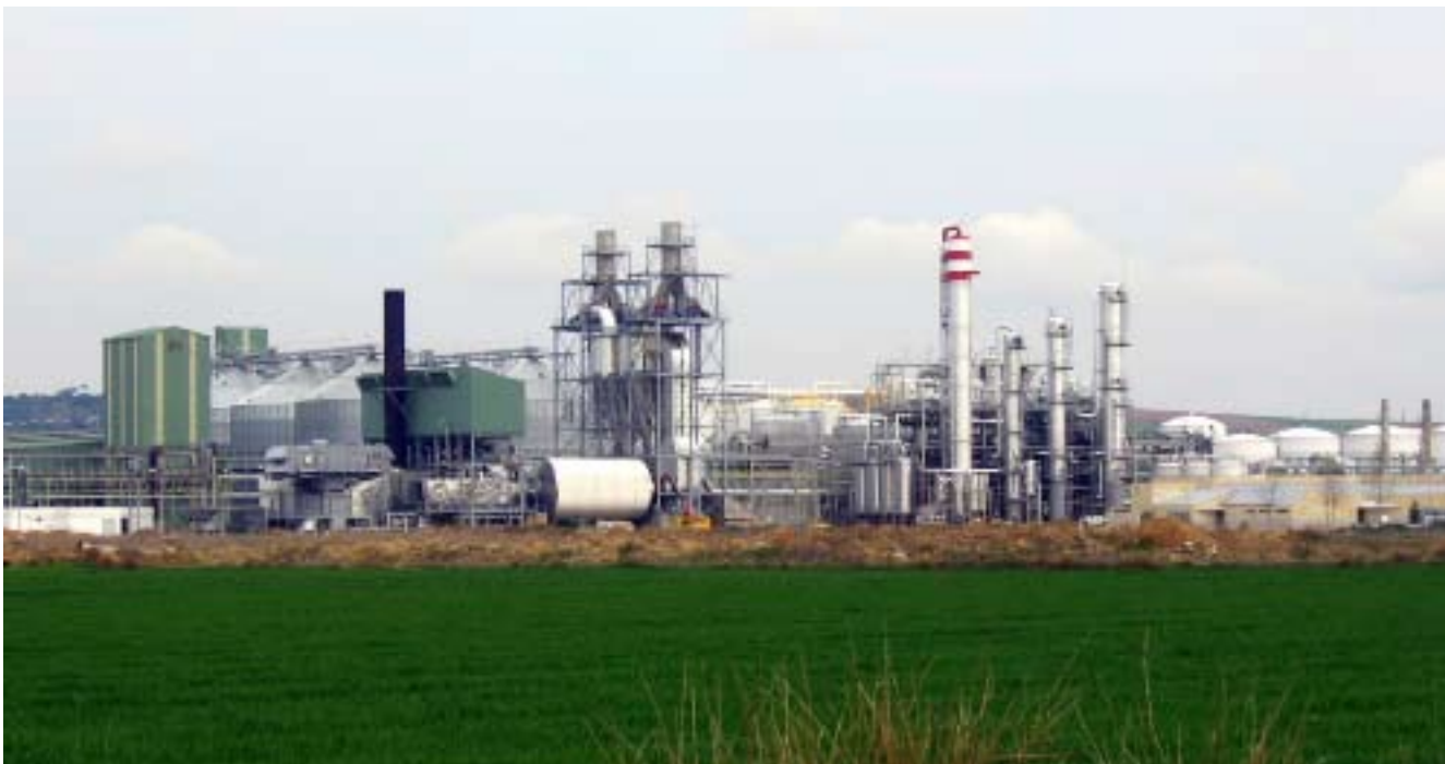
Bioethanol plant in Babilafuente, Salamanca
