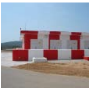
Moving of VOR regulator rooms at Ibiza Airport
