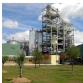
Biomass-to-bioethanol plant in Babilafuente, Salamanca
