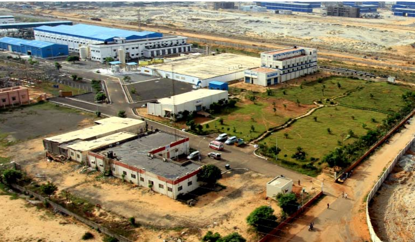
Shot of the Chennai desalination plant (100,000 m 3 /day) in production since July 2010
