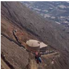
Drinking water and sewerage systems commissioned by Sedapal for the areas of Pariachi, La Gloria, San Juan, Horacio Zevallos and annexed territories.
