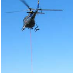
Pilot high-voltage line stringing by helicopter in Spain
