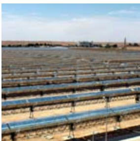
SPP-1 (Hassi R'Mel, Algeria)
