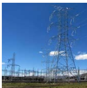
TL concession, Carhuamayo, Paragsha, Conococha, Huallanca, Cajamarca, Cerro Corona, Carhuaquero 220 kV TL Conococha – Kiman Ayllu L4 Norte – Arrival at the Cajamarca Norte substation, Peru
