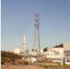
Enernova cogeneration plant in Ayamonte (Huelva)
