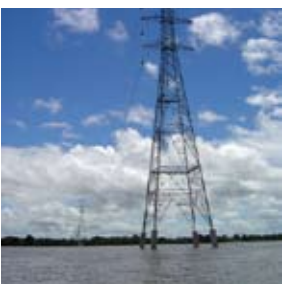
500 kV transmission tower, ATE III Itacaiúnas (Pará)-Colinas (Tocantins)
