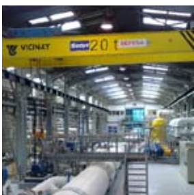
Production facility at the Skikda desalination plant (Algeria)
