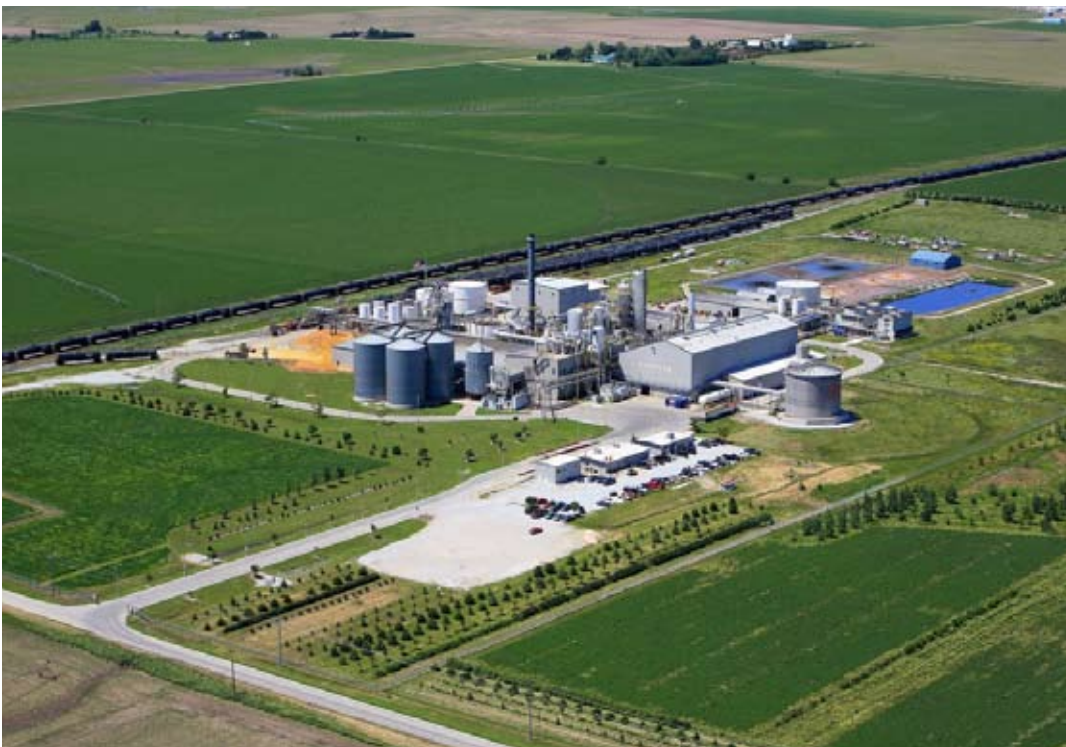
Second generation ethanol production plant in Salamanca, Abengoa Bioenergy
