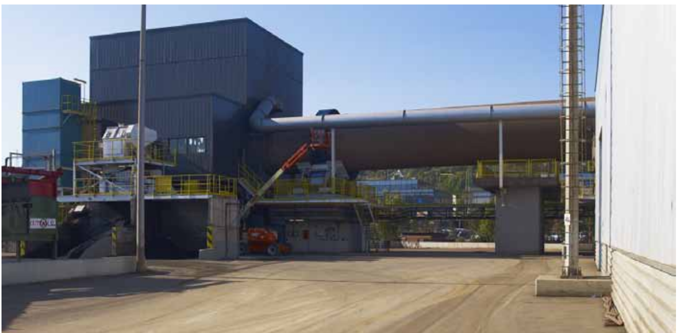
Side view of the Waelz furnace at Befesa Zinc Aser facilities, Spain
