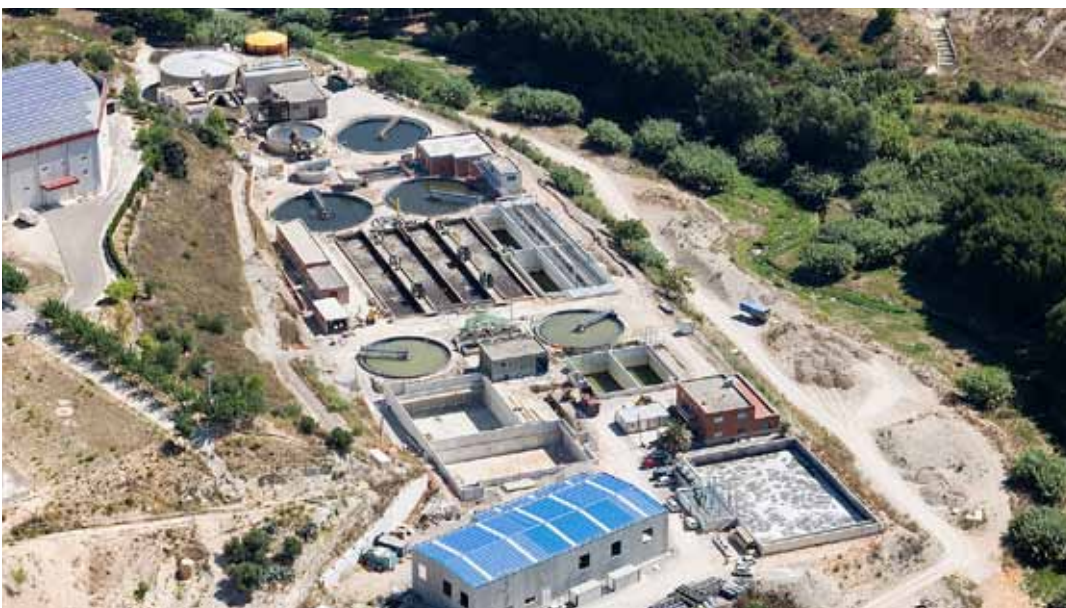
View of the Alcoy WWT plant, Spain
