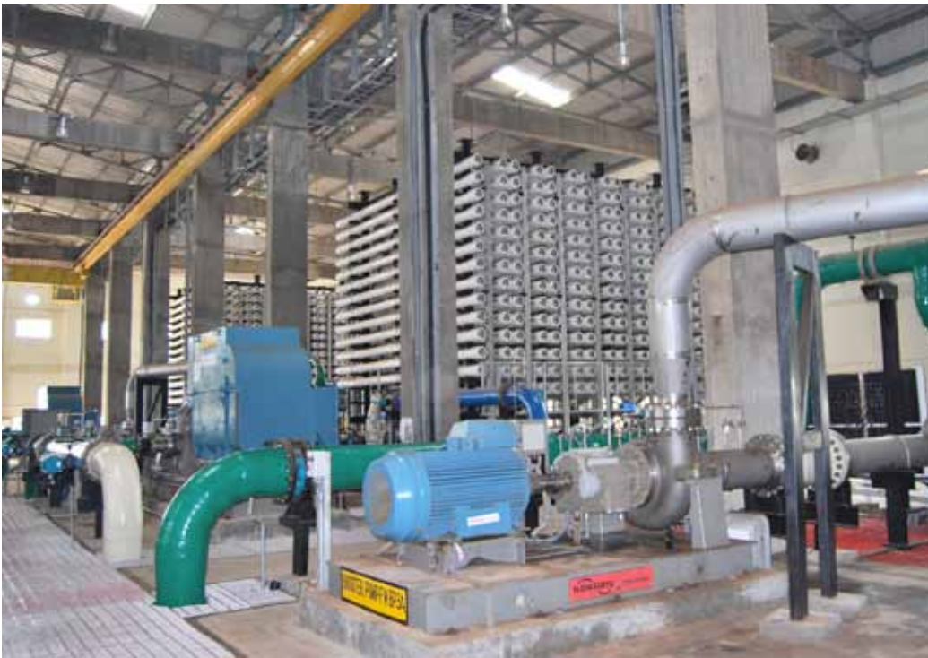
Membrane frame and other equipment at the Chennai desalination plant, India
