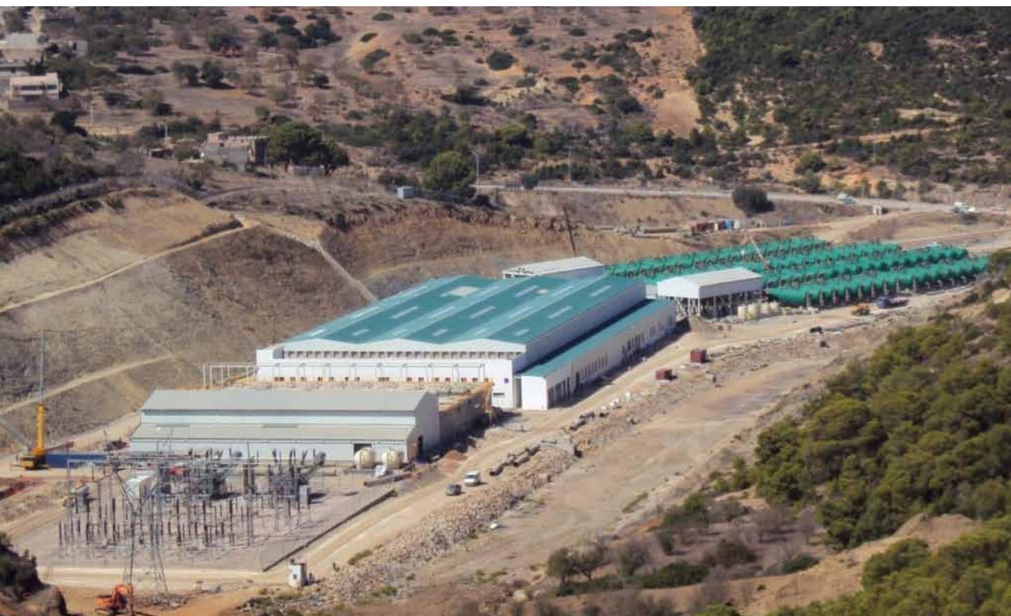
View of the Honaine desalination plant under construction, Algeria
