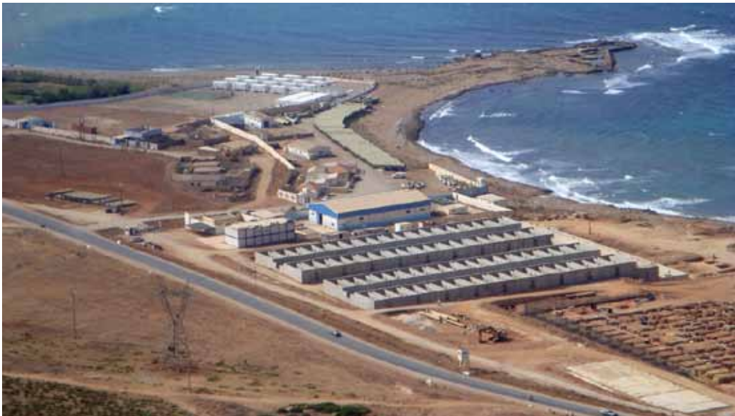
View of the Tenes desalination site, Algeria
