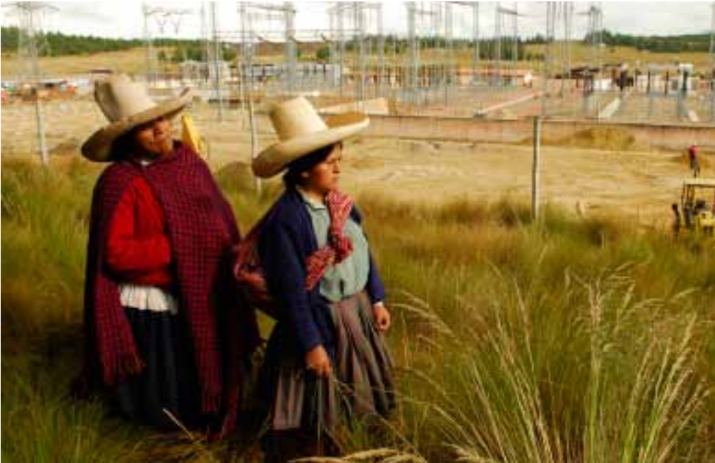
Peasants next to the Cajamarca substation on the 220 kV Carhuamayo-Carhuaquero transmission line in Peru
