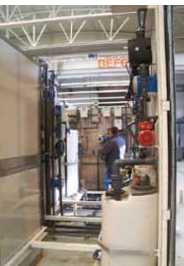
MBR pilot plant
