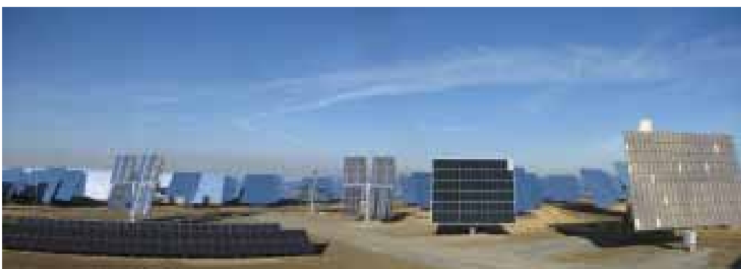
Different concentrating photovoltaic systems
