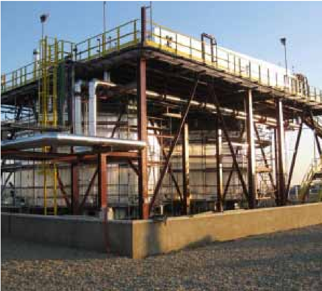
Molten salt storage pilot plant, operational since 2009 at the Solucar platform, Seville
