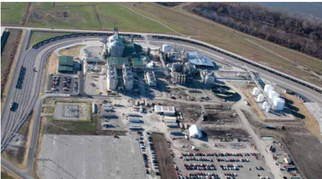
Bioethanol plant in Madison, Illinois
