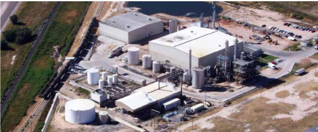
Bioethanol plant in Portales, New Mexico
