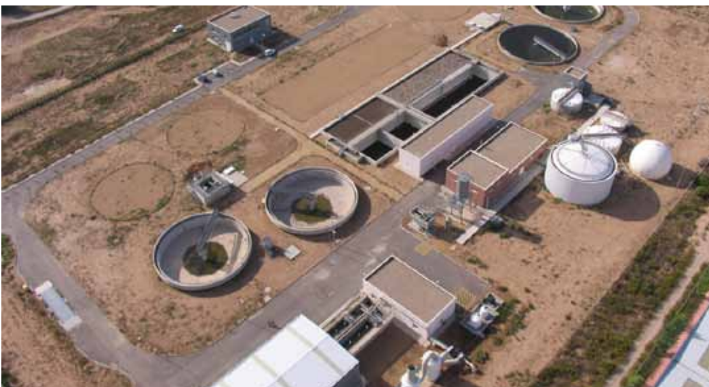
Aerial shot of the Meco treatment plant, Spain
