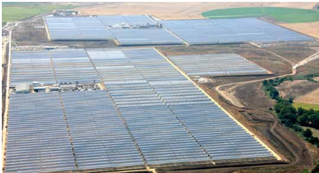
Solnova 1, Solnova 3 and Solnova 4 solar trough collector plants in operation at the Solúcar complex Seville
