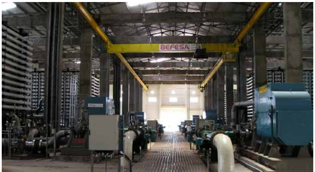
Inside the Chennai desalination plant, India
