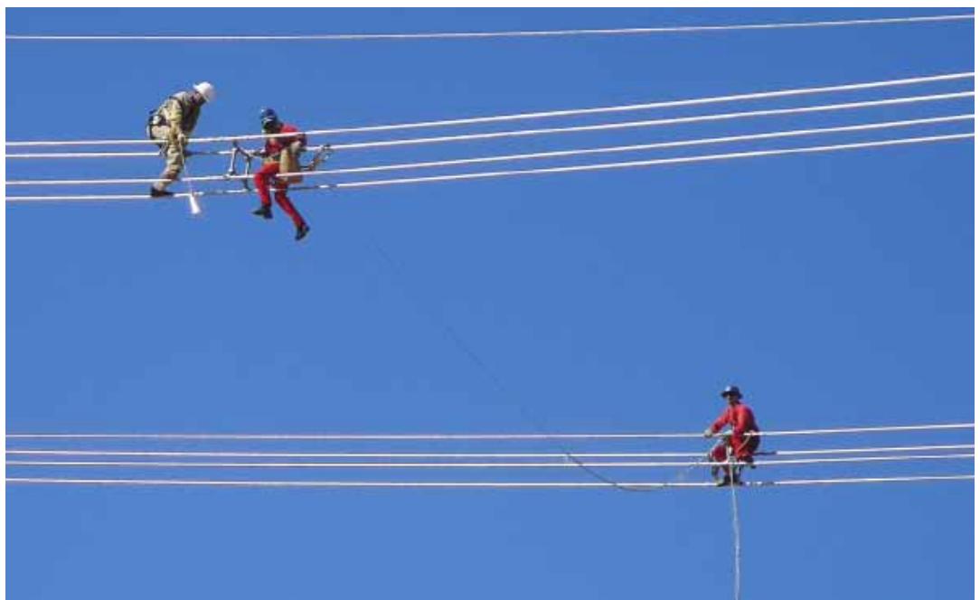
Abengoa Brasil employees carrying out O&M work on a power transmission line
