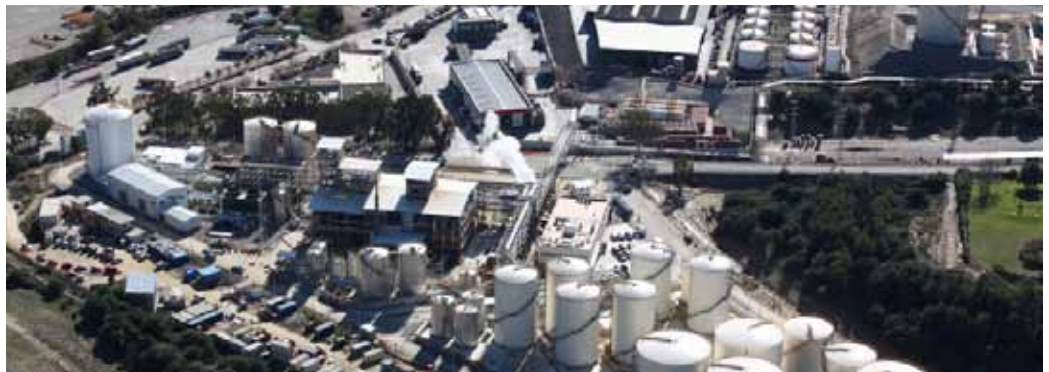
Biodiesel plant in San Roque, Cadiz
