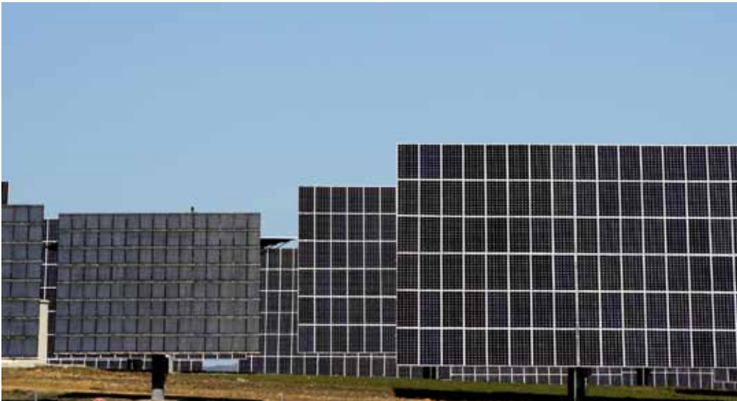
Photovoltaic plant comprising conventional and high-concentration heliostats operating at the Solúcar complex in Seville
