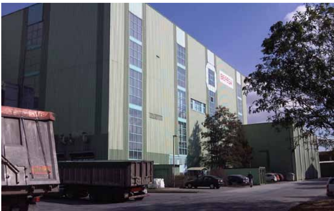
View of the main Befesa Salzschlacke building in Hannover, Germany
