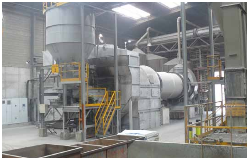
Aluminum swarf dryer at Befesa Aluminio facilities in Las Franquesas del Valles, Spain
