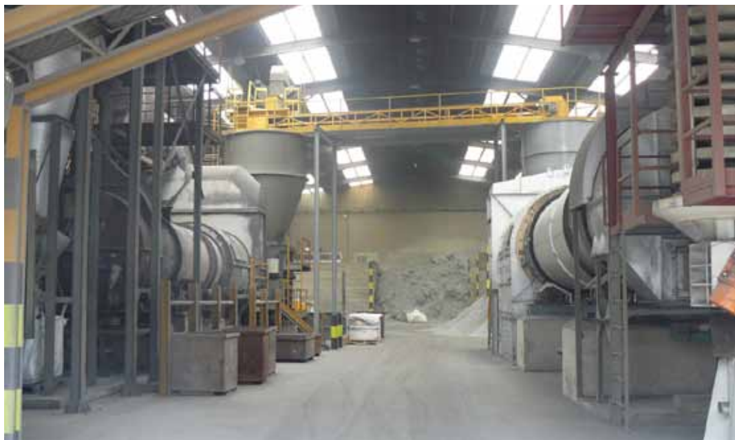
Aluminum swarf dryers at Befesa Aluminio facilities in Las Franquesas del Valles, Spain
