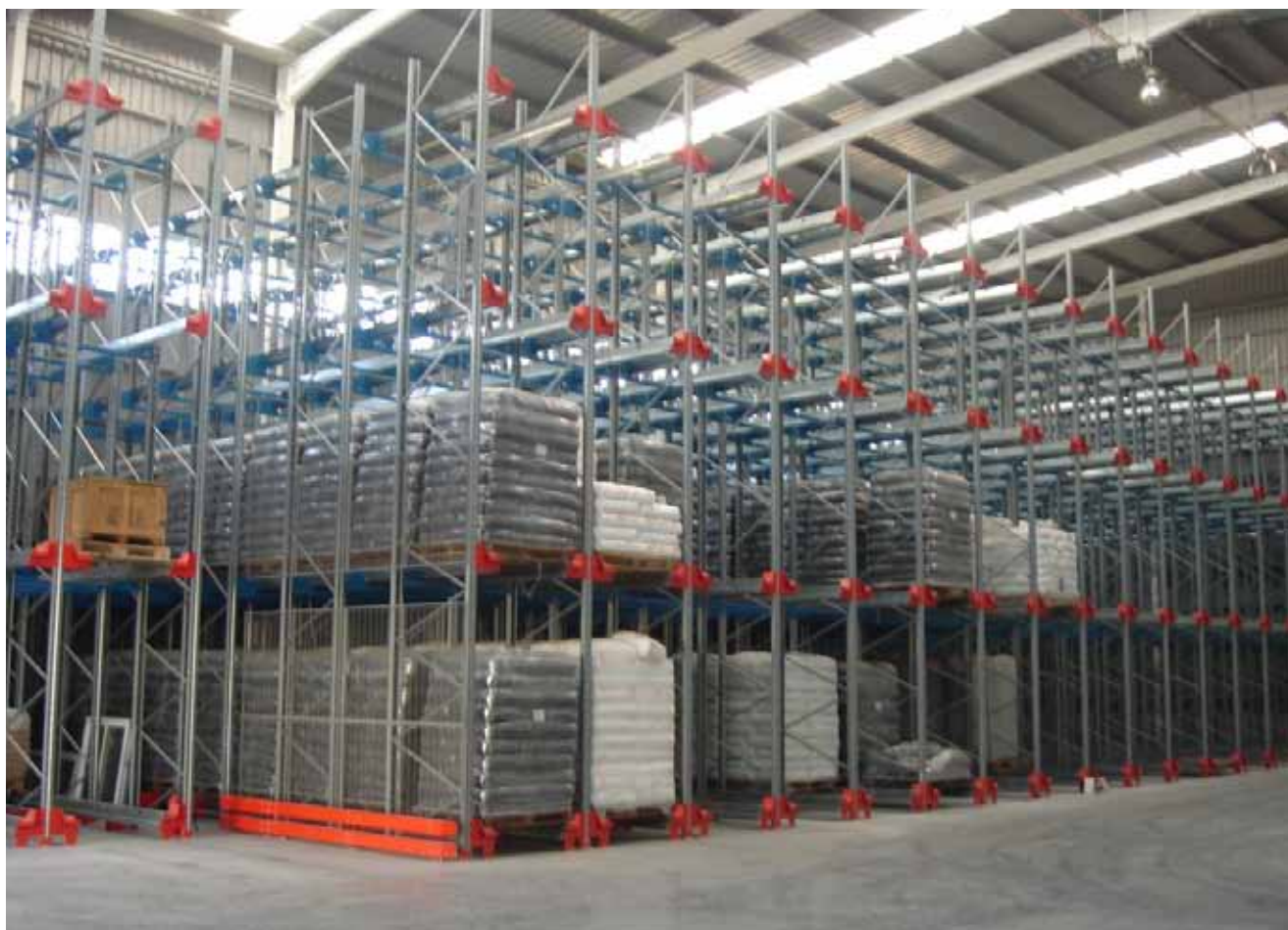
Raw material and end product storage facility at the new Befesa Plásticos plant, Spain
