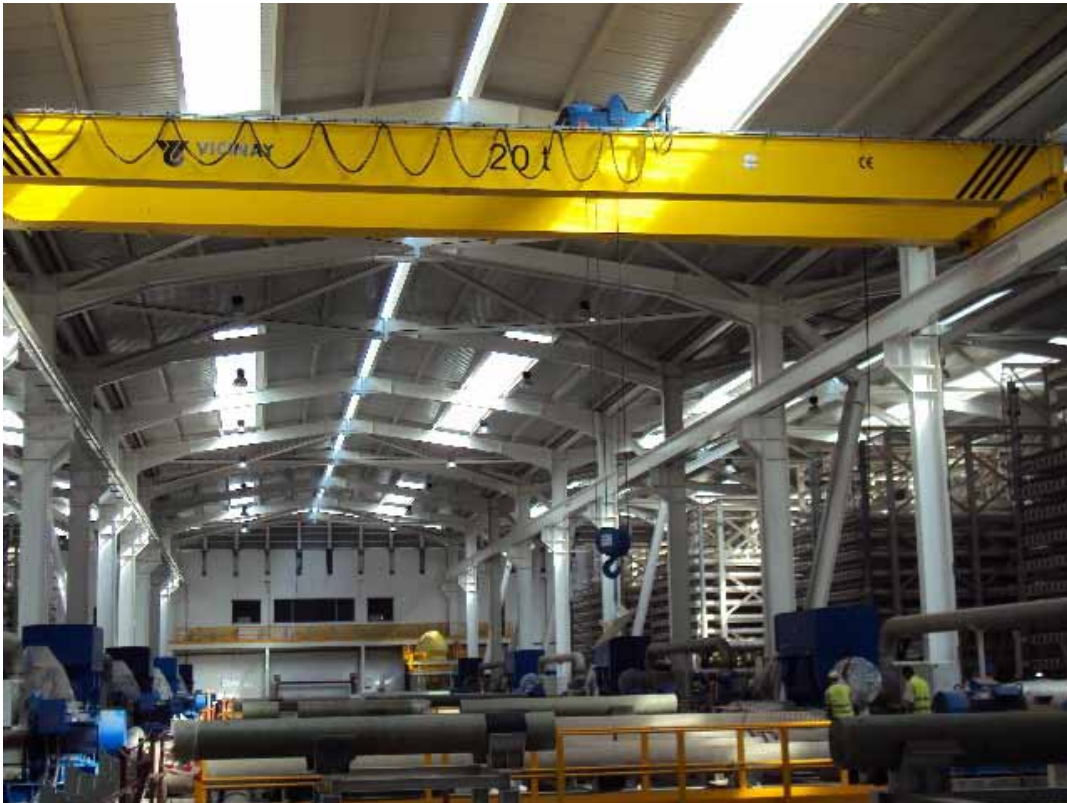
Inside the Honaine desalination plant under construction, Algeria
