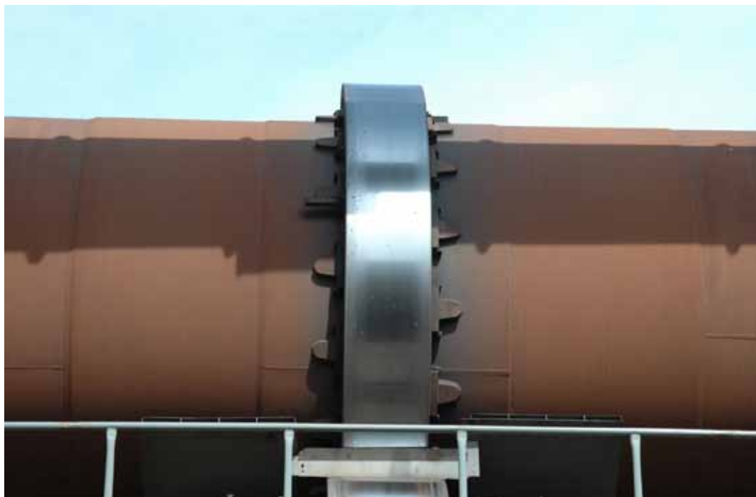
Waelz furnace at Befesa Zinc Freiburg facilities, Germany
