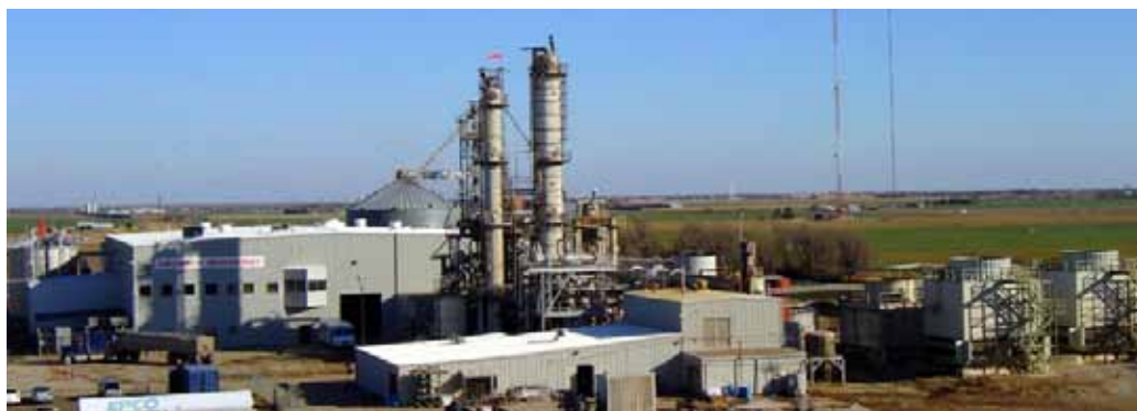
Bioethanol plant in Colwich, Kansas
