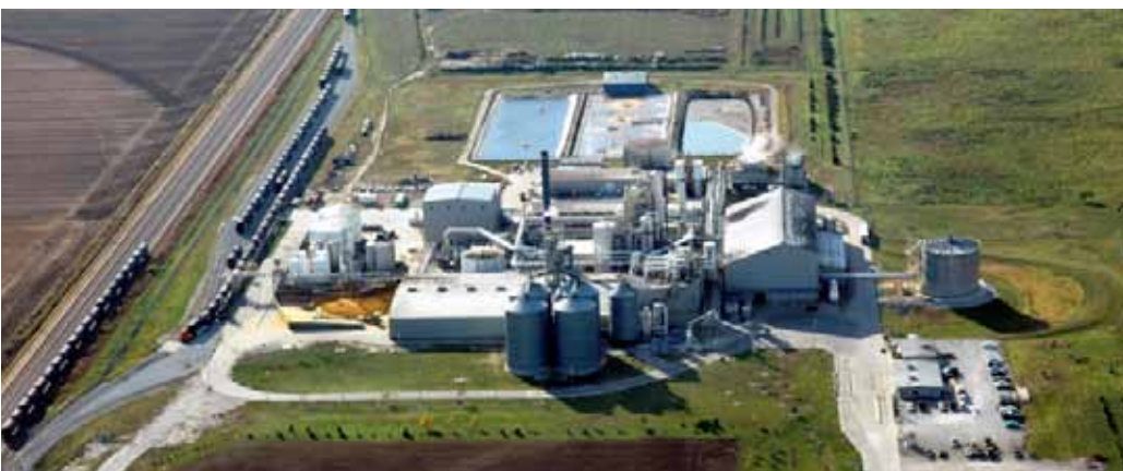
Bioethanol plant in York, Nebraska
