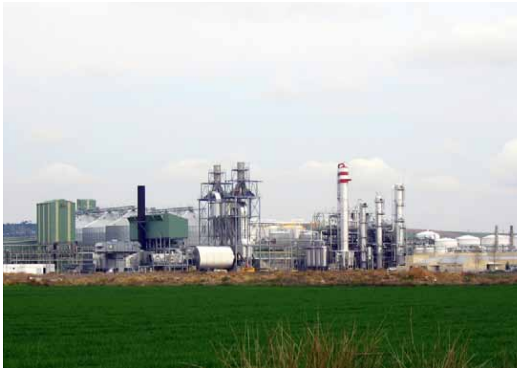
Bioethanol plant in Babilafuente, Salamanca
