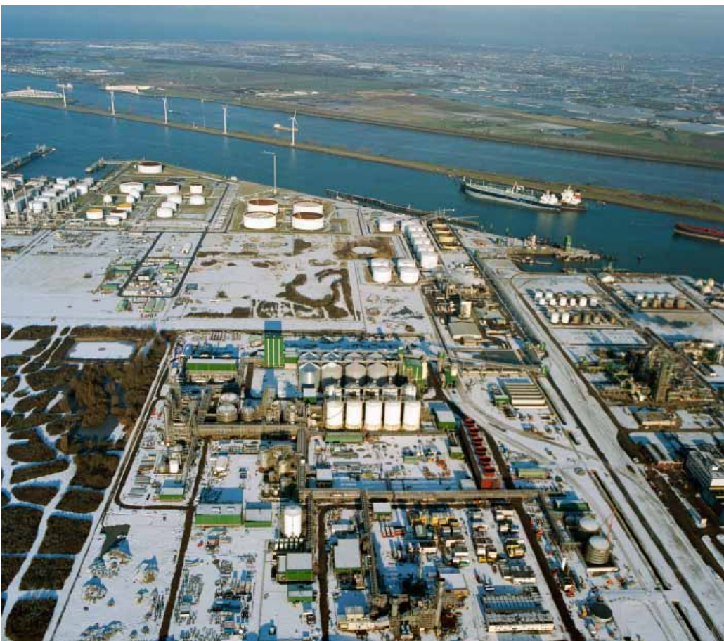
Bioethanol plant at the Europoort, Rotterdam, the Netherlands
