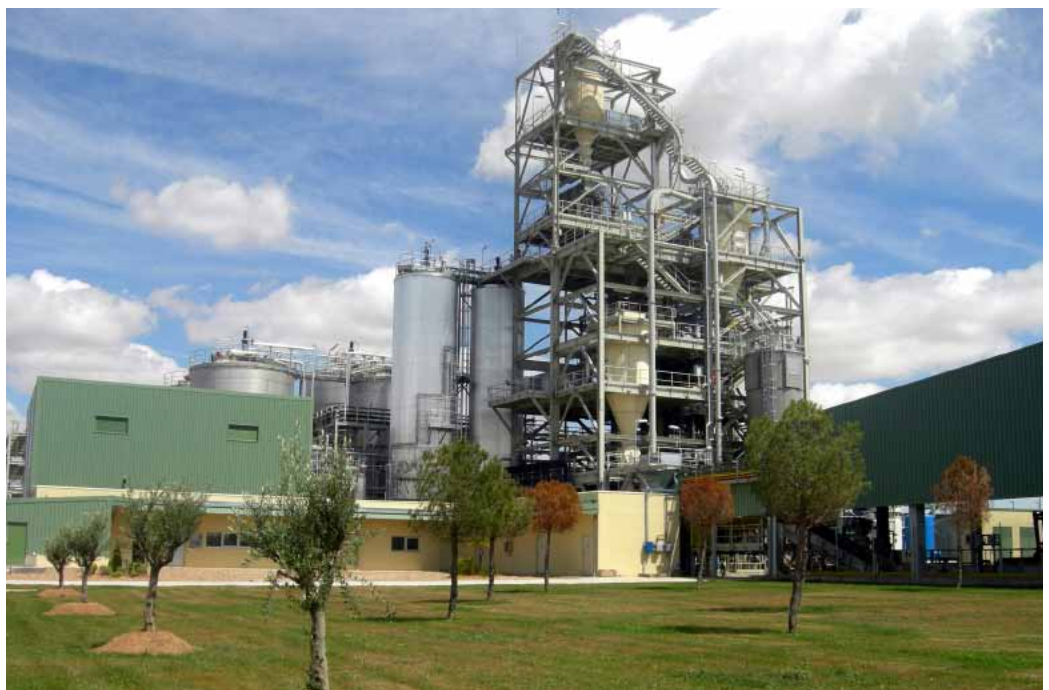
Biomass-to-bioethanol plant in Babilafuente, Salamanca
