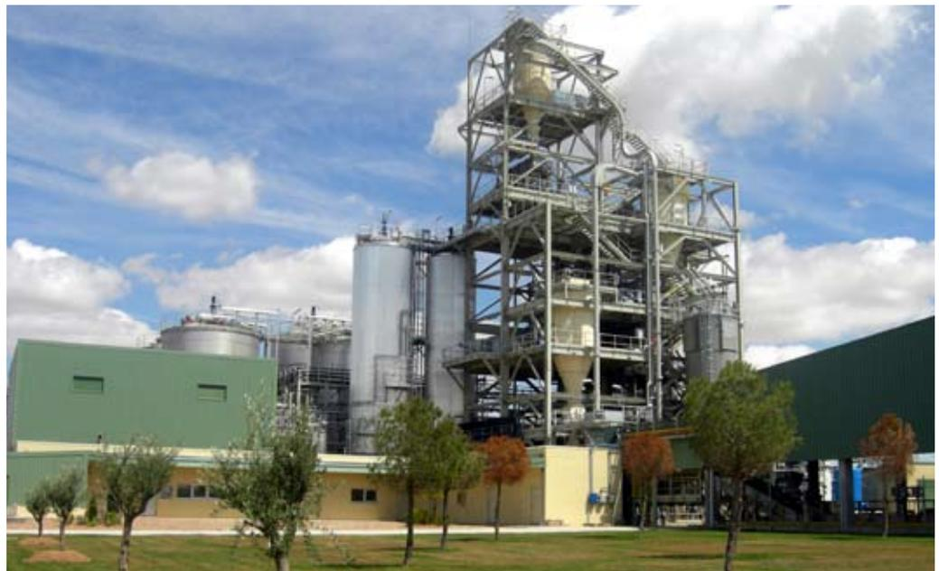
Managed by Abengoa Bioenergía Nuevas Tecnologías, the biomass plant was completed in December 2008 and has been fully operational since September 2009. It is the world's first plant to utilize this technology on such a scale. It is located within the Biocarburantes de Castilla y León plant, meaning that both facilities share common services and process chains. The ethanol it produces is distilled to 42 % and then concentrated and dehydrated.
