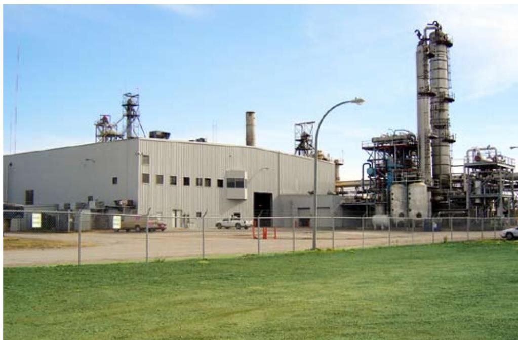
One of the three operational plants fully owned by Abengoa Bioenergy Corporation in North America. The plant currently operates at 100 % capacity and continues to report excellent efficiency and consistent operations. Production capacity amounts to 25 Mgal per year, achieved through continuous batch cooking and fermentation processes. The CO<sub>2</sub> generated is captured and refined by an on-site client and the plant currently employs 48 highly qualified workers.
