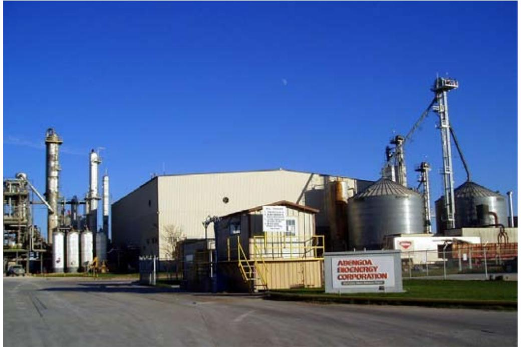
Expansion work was completed in 2006 to double production capacity by utilizing batch cooking and fermentation processes, with two separate distillation and dehydration stages. The DGS produced is not dried in the process and 100 % of the co-product is sold in its natural state. The plant can operate with corn and sorghum simultaneously. Bioethanol production capacity stands at 27 Mgal per year and the plant currently employs 48 highly qualified workers.
