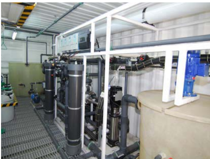
Befesa Water. High-efficiency reverse osmosis desalination pilot plant
