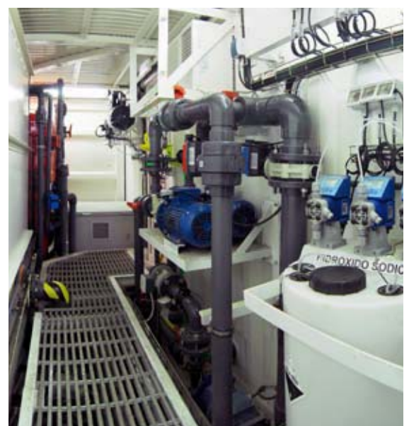
Befesa Water. Advanced pre-treatment systems pilot plant.
