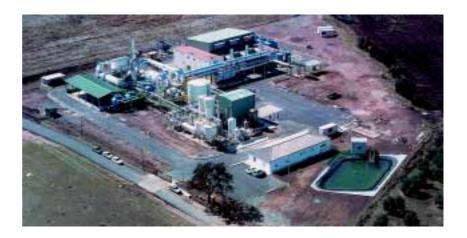
Extension of the Barranco Seco II wastewater treatment plant (Las Palmas) for the Spanish Environment Ministry, serving a population of 245,000. It operates on the basis of tertiary treatments using electrodialysis reversal (EDR) to provide 26,000 m3 of water a day for irrigation purposes.
