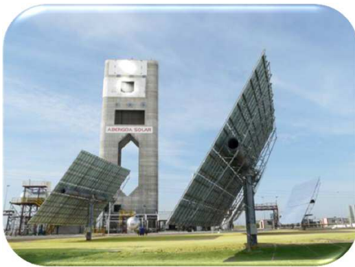
Superheated steam “Eureka” pilot plant
