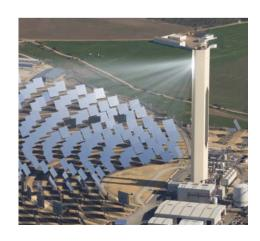
**Operating principle:** A circular array of heliostats (2 axis tracking mirror) is used to concentrate sunlight to a central receiver mounted on the top of a tower. A heat transfer medium in this receiver absorbs the highly concentrated radiation and coverts it into thermal energy to be used by a turbine.
