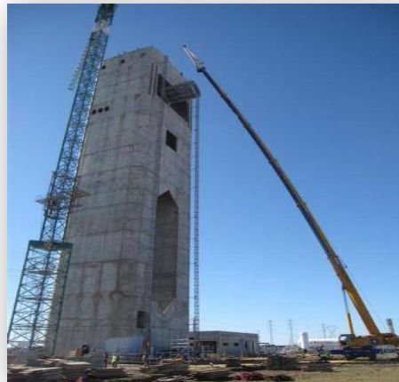
Solugas Pilot Plant
