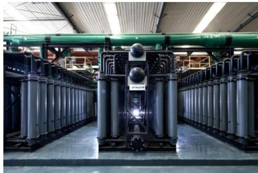
UF membrane racks in Qindao desalination plant
