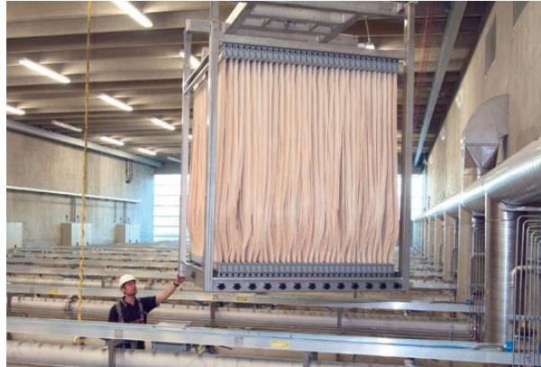
Worker installing hollow fiber membranes in MBR
