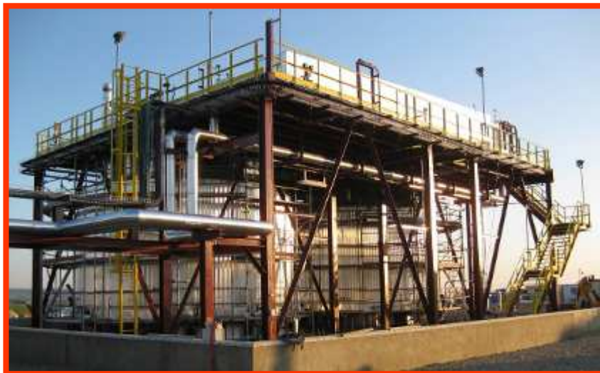
Demonstration plant located at the company's Solucar Platform in Spain
