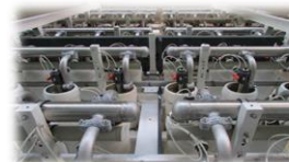
Membrane lab Water (Bilbao, Spain)
