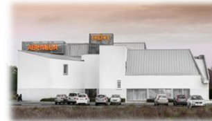
R&D center Water (Seville, Spain)
