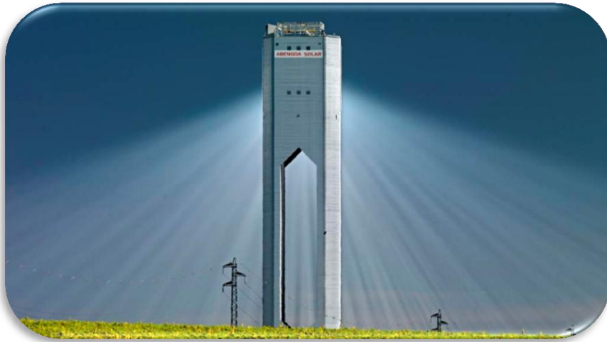
20 MW CSP Tower (Spain)
